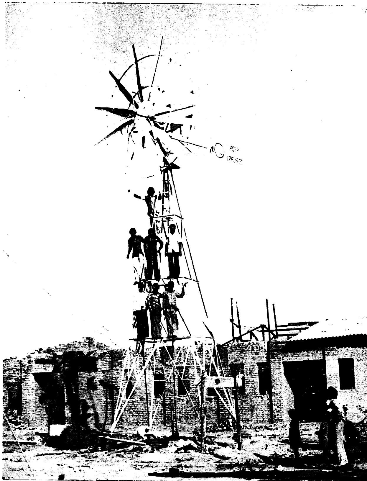
A 12 PU 500 -windmill being installed for drinking water supply (February 1980, Gohri near Allahabad, U.P. India).
