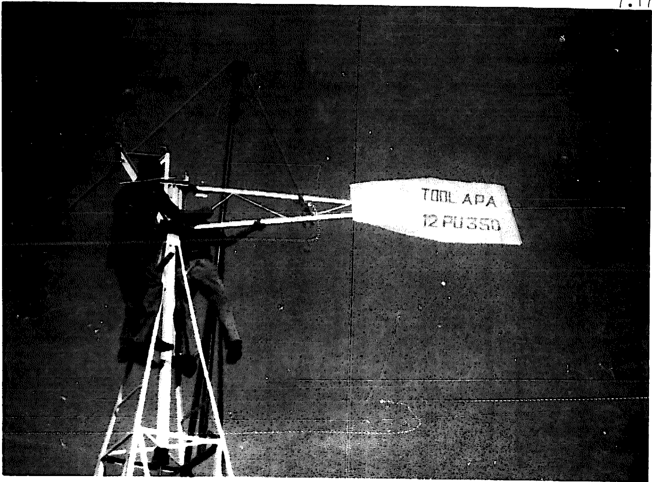
Installing a 12 PU 350 head construction
