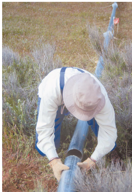
Above: NRG tower sections slip fit together and seat firmly when the tower is raised.
