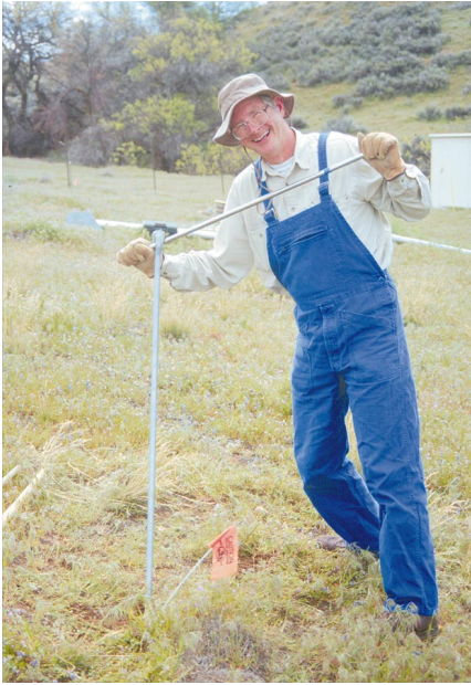
Above: The screw anchors can be driven by hand.
