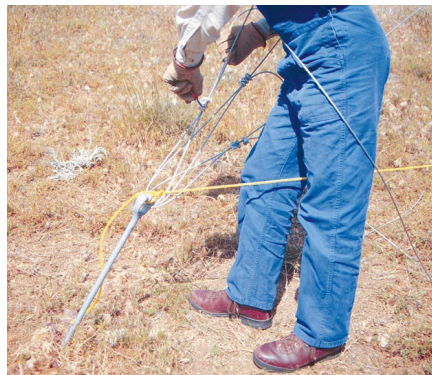
Above: Adjusting cable tension. The NRG tower system doesn't use turnbuckles which allows for quick adjustments under less than ideal site conditions.
