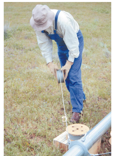
Below: Unreeling the guy cables. All attachments to the guy bracket are swaged, simplifying assembly.
