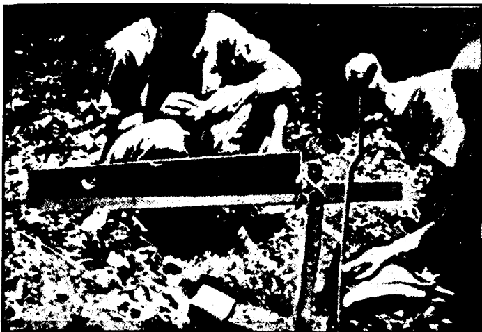
With the straightedge held level, vertical height between a pair of pegs is read off and noted.
