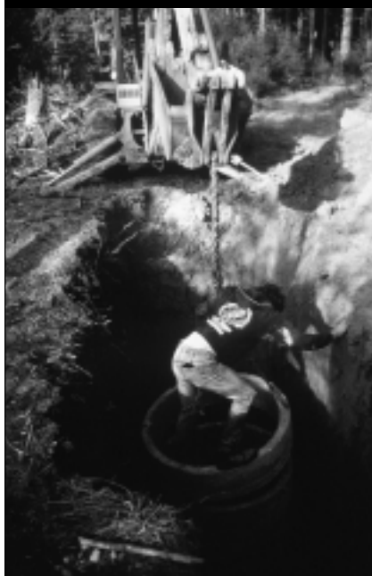
A shallow well may be dug with a backhoe.
