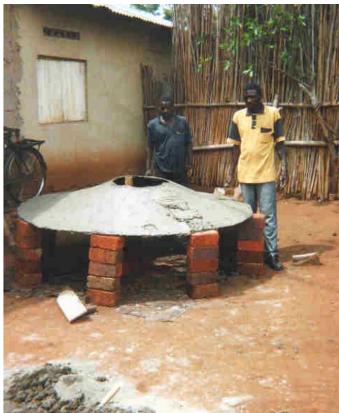
Figure 10 – 6mm steel framework being formed by local masons in western Uganda for the TSF tank cover.
