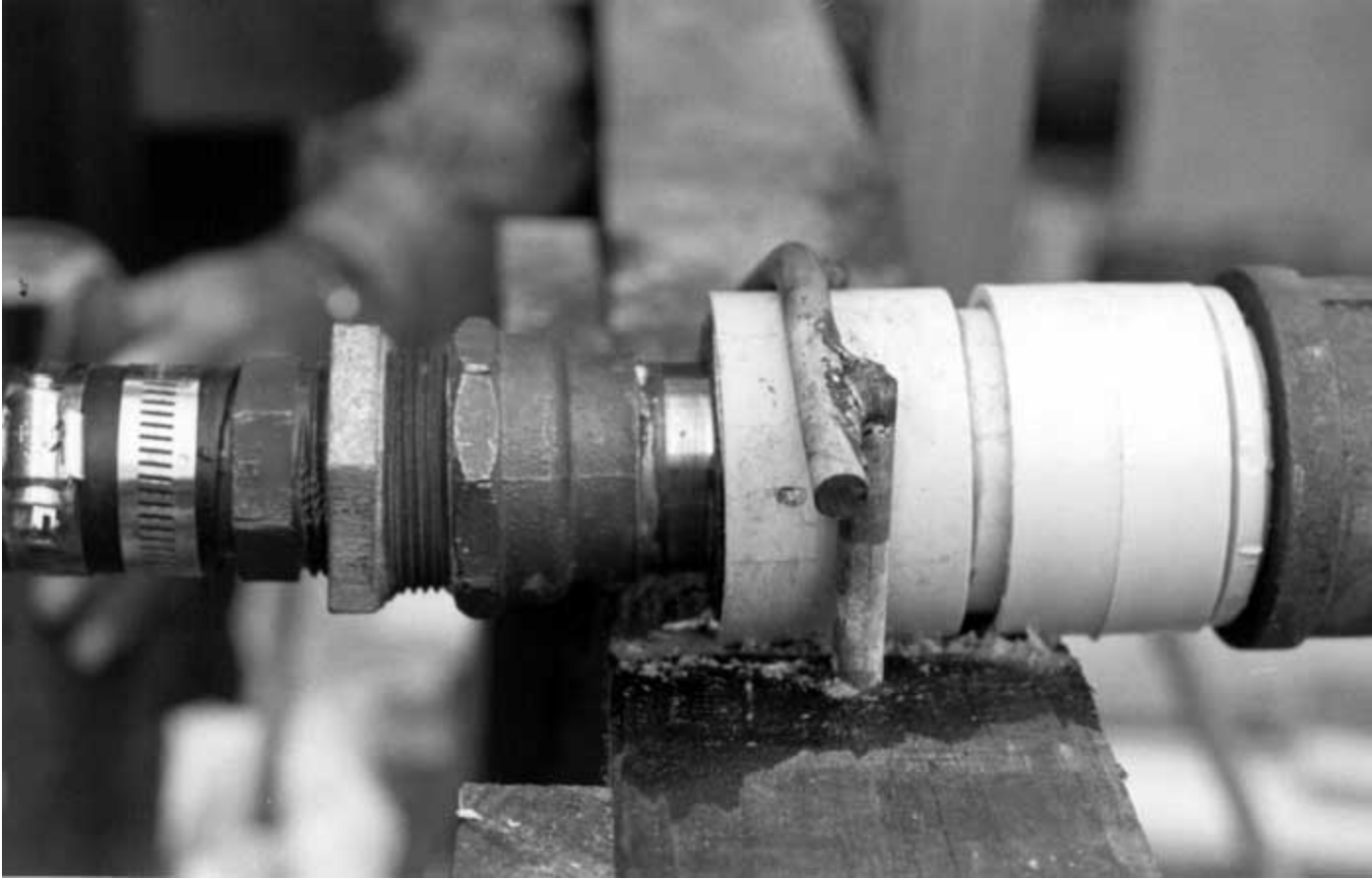
Figure 5: Close-up of rotary fitting
