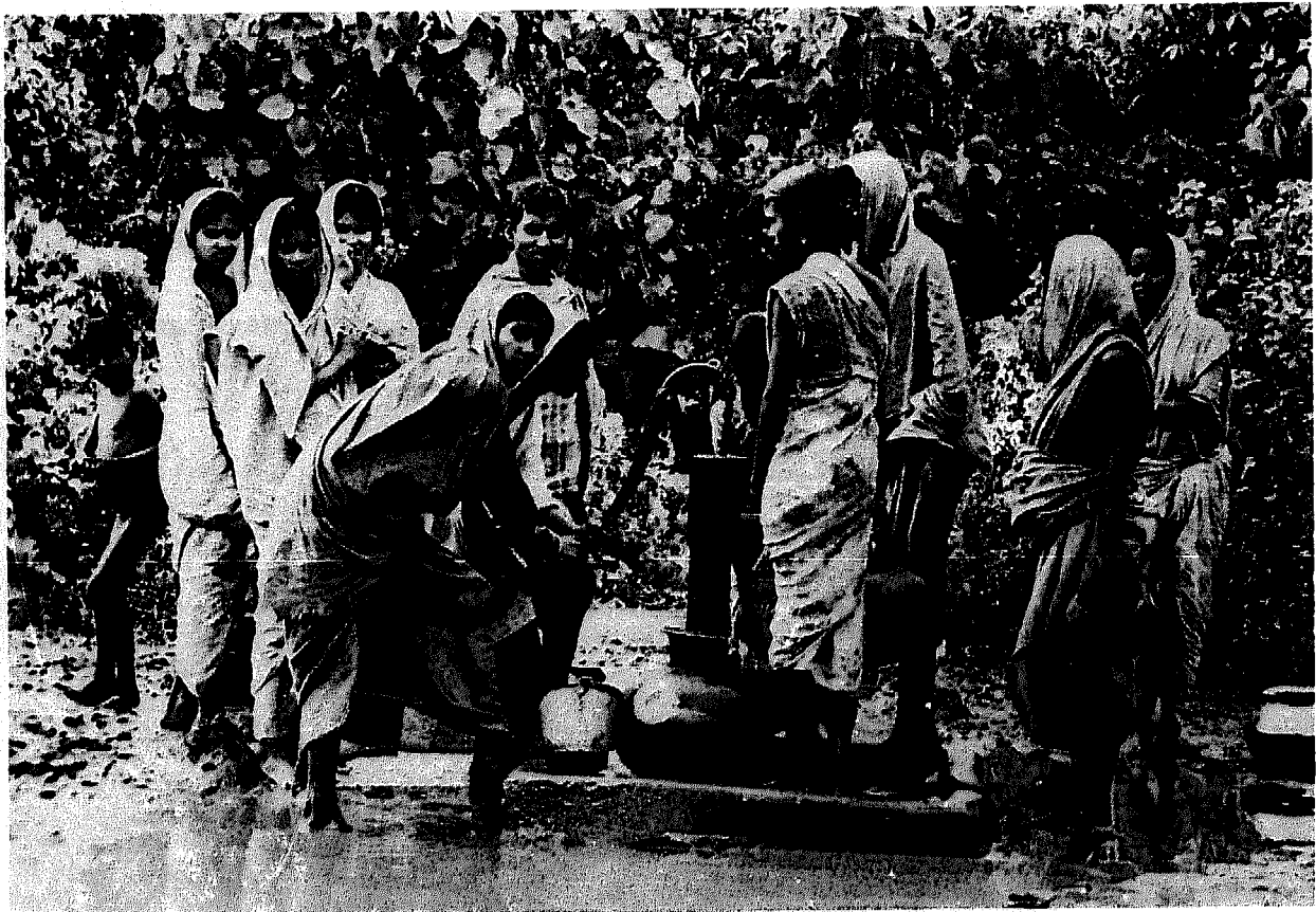
FIGURE 4-3 HAND PUMP WITH INADEQUATE DRAINAGE
