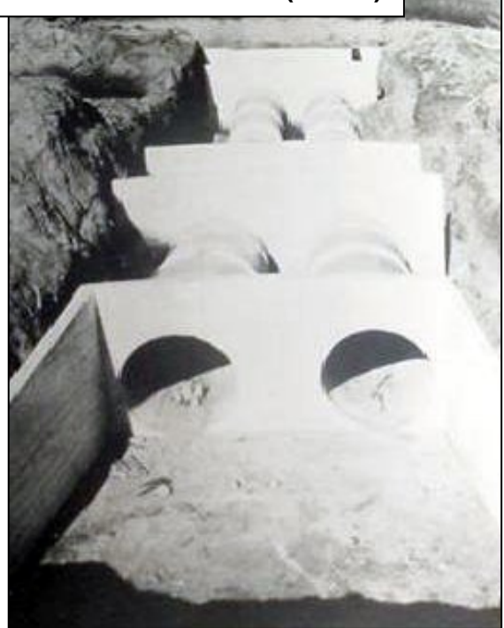
Culvert with collars (USBR)
