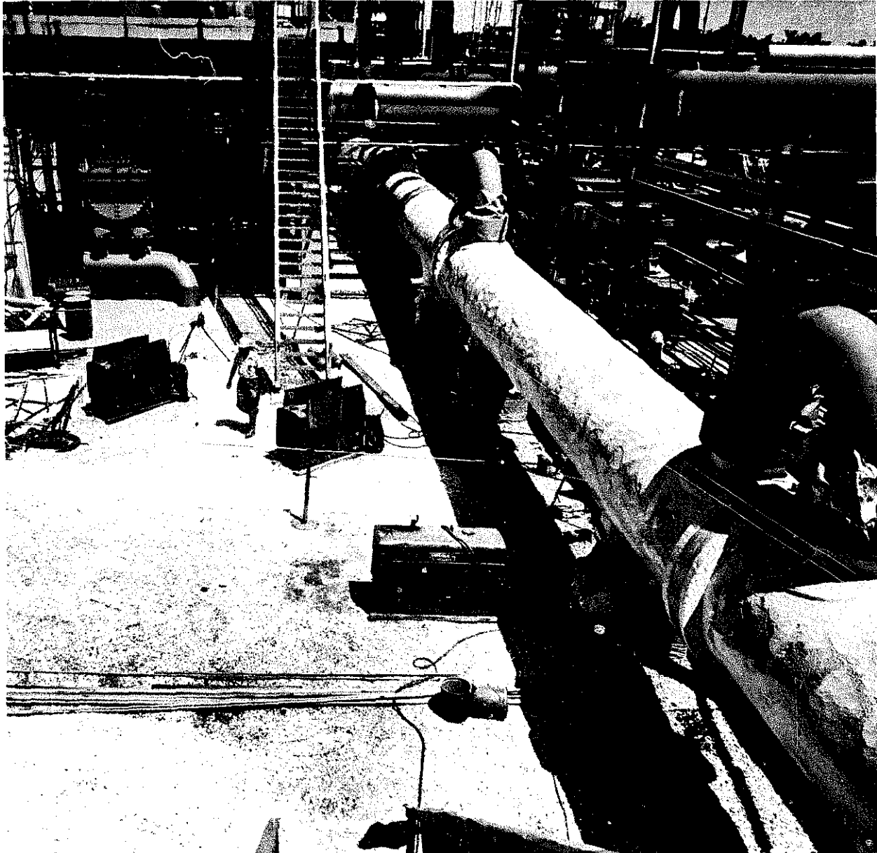
Typical example of welded high pressure pipe in a gas processing plant. Note the engine driven welding machines.
