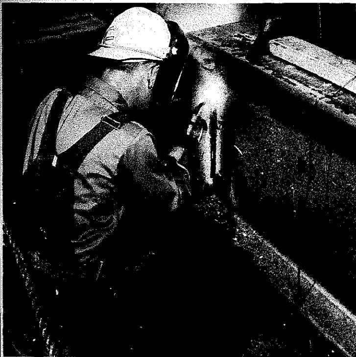
Fig. 5-8. Before all-position electrodes for self-shielded flux-cored arc welding were developed, beam web-to-column connections in building erection were made with stick electrodes. If the flange-to-column joints were made with semiautomatic equipment, the operator had to change to the stick electrode for the vertical joint, or the connection had to be made by bolting the web to an angle welded to the column. The all-position electrode wires were the development that made possible one-process mechanized welding in building erection, with all of its incidental benefits in the scheduling of erection operations.
