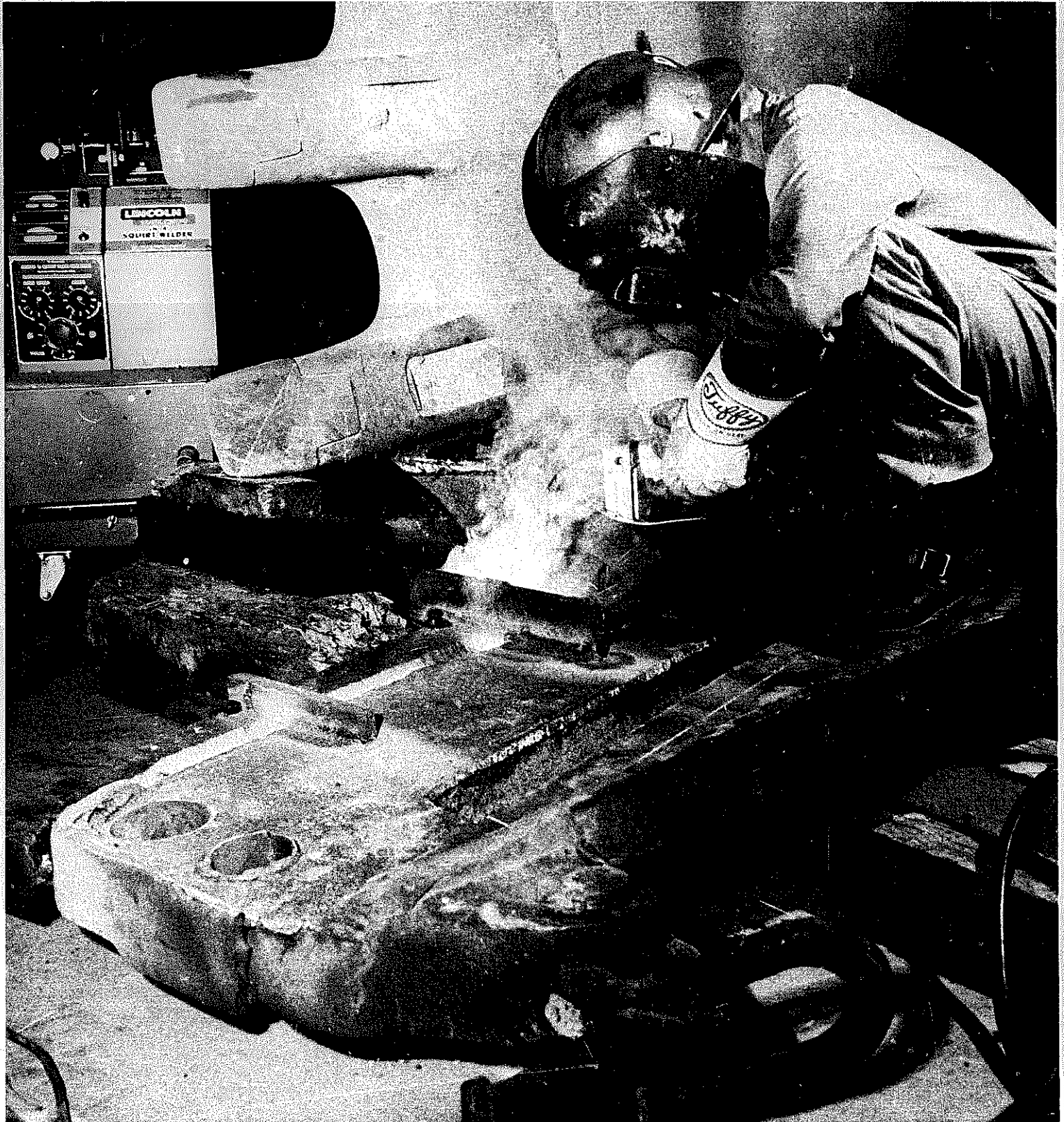
The lip on a dragline bucket wears thin and must be repaired. Here the worn areas were cut out and replaced with new plate. The patches are being welded in with a semiautomatic process.
