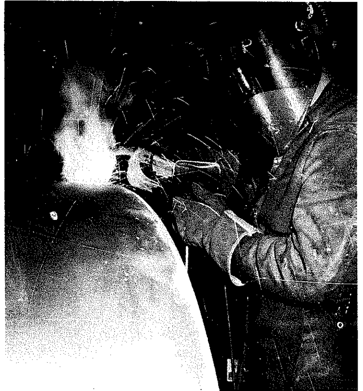
Fig. 4-32. The fixturing equipment being used with the semiautomatic welding gun here in the welding of a head to a cylinder for a storage tank takes the work even a step further than the fixture in Fig. 4-31 toward full mechanization. A roller mechanism is being used to turn the cylinder under the gun, and the weldor's hand rests on a support so he can hold the gun precisely in reference to the centerline of the cylinder.
