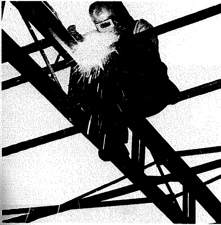
Much of the welding done in building construction is the shielded metal-arc process.
