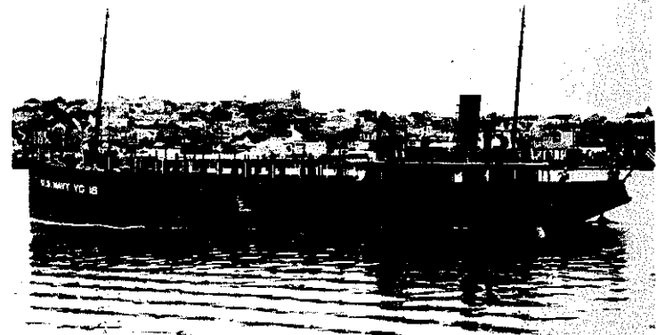
Fig. 1-6. An all-welded naval vessel that won a major award in a design competition in 1932.
