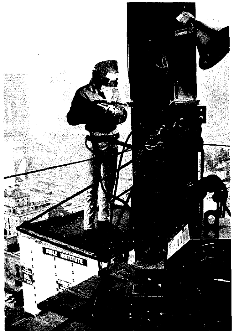
Fig. 1-14. Splicing a column during the erection of a building in Los Angeles, using the semiautomatic self-shielded, flux-cored arc-welding process.
