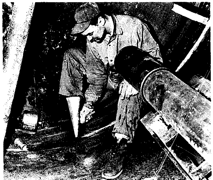
Fig. 1-10. Four passes are made inside the tower in this flame-gouged seam joining the head to the shell. A current of 400 amperes and a speed of 14 inches per minute are used. The absence of smoke, spatter, and visible arc rays increases operator efficiency in applications in close quarters such as this. Welds deposited are dense and free of hydrogen, which reduces the tendency to cracking and eliminates porosity. The weld must pass X-ray examination.
