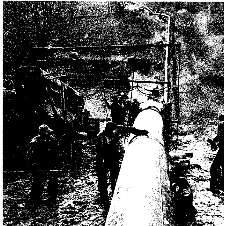
The stick-electrode process does an excellent job field welding pipe, sometimes under adverse conditions.
