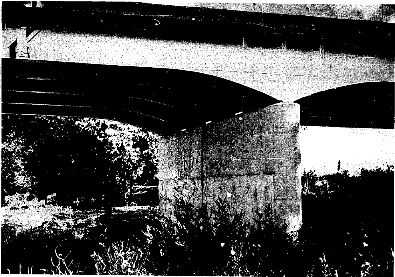
Bridge girder design with a hinged connection.
