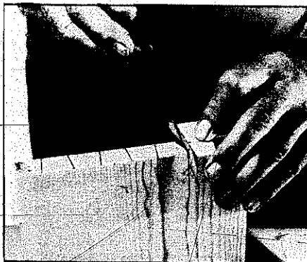
Use a template for marking end cuts when many dovetails are required.
