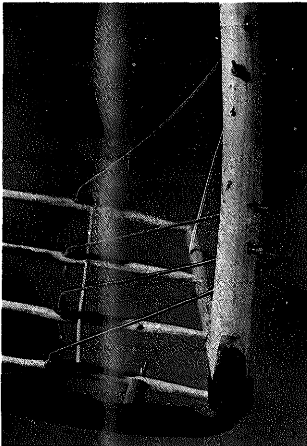
The supporting all-thread strut is bolted in place with a wing nut.
