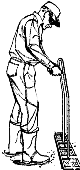
Fig. 31.6. A tamper. Tamping newly placed concrete forces the large aggregates below the surface and brings mortar to the surface for finishing.
