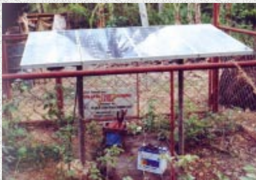
Two-outlet self-regulating SBCS
