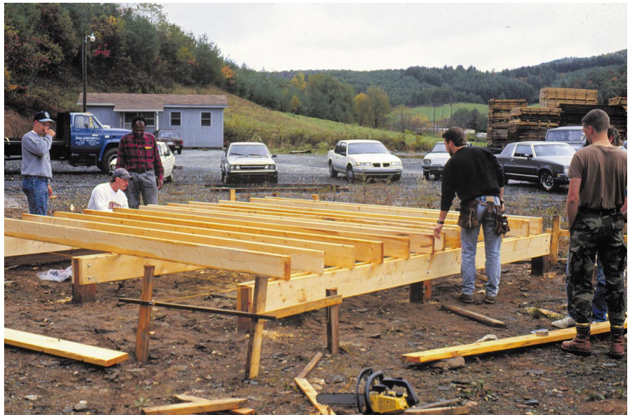
Above: Laying out foundation and floor.
