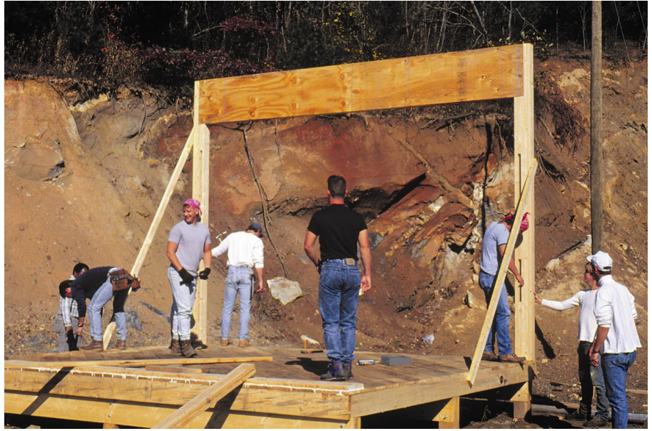
Above: Bracing the north wall.
