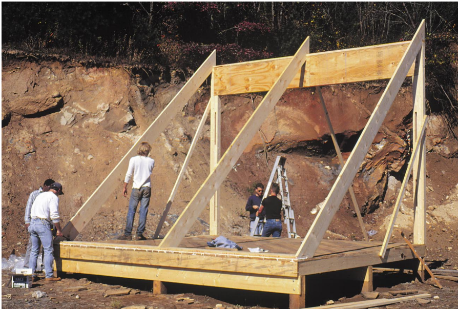
Above: Setting up 2 by 12 south wall rafters.
