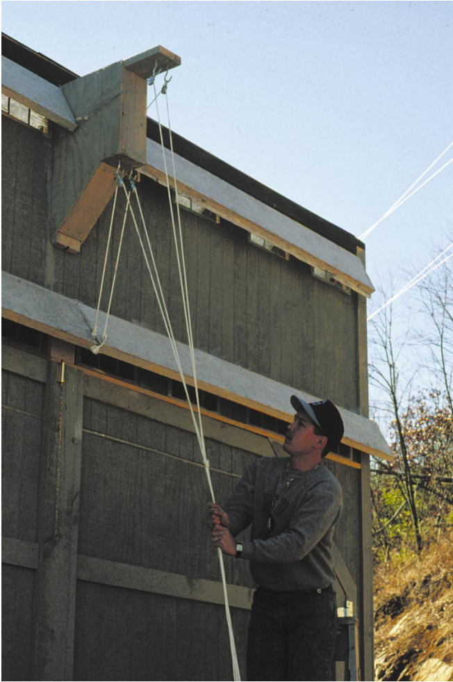
Above: Setting up vent control lines.
