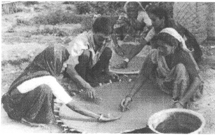
Figure 5. The surface is being smoothed and then left for drying for 1 day.
