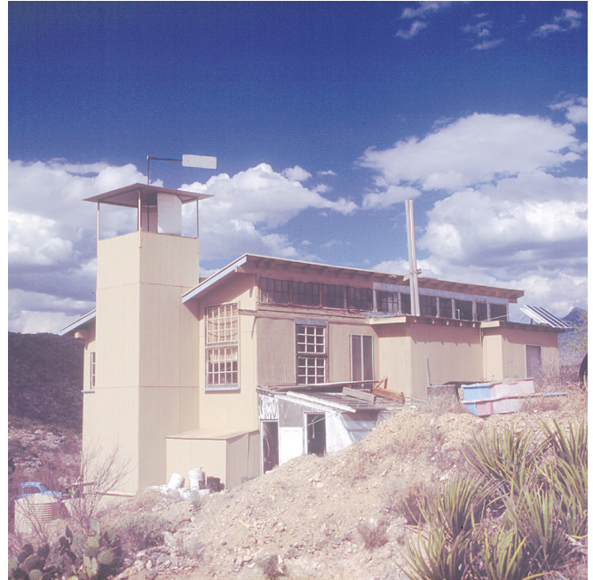
Above: The upwind scoop on the cool tower guides hot dry air past the wet pads. Water evaporates, and the moist cool air drops down inside the house. Downwind scoops on the roof exhaust warm air.
