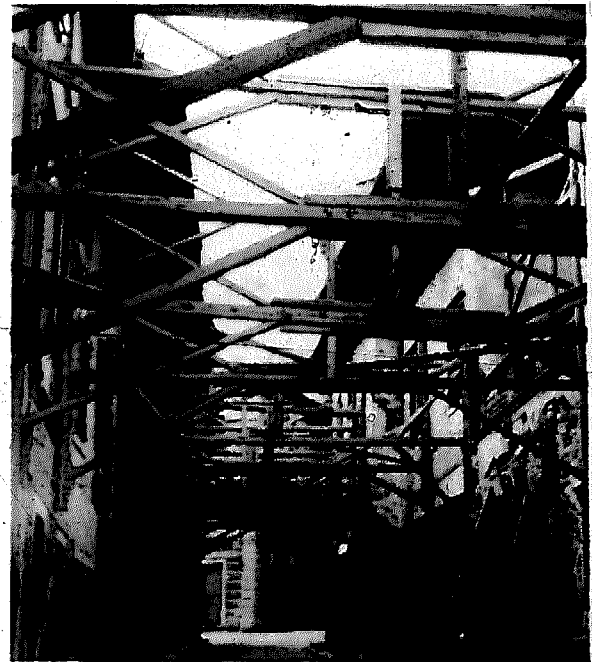
73 Gemona, Italy. Wooden shoring to support the facades of the historic town prior to reconstruction. But this all collapsed in the second earthquake, September 1976
