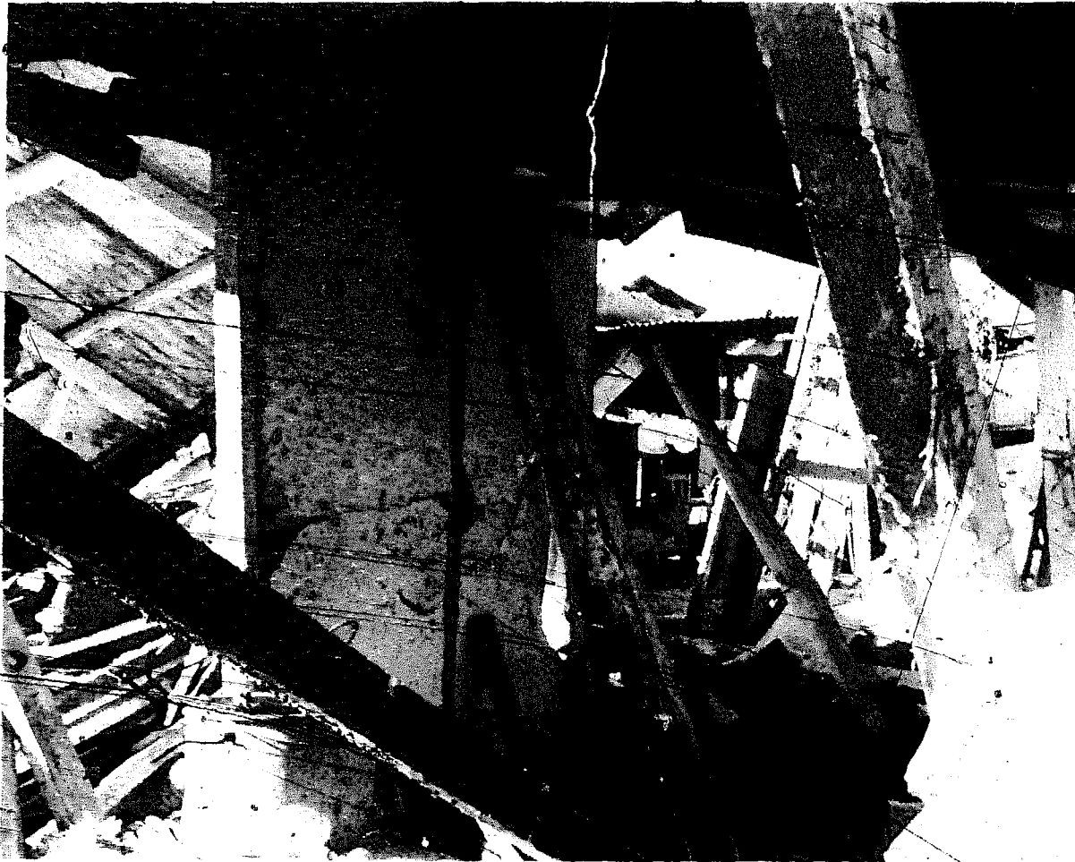
15 Housing in Guatemala city, showing badly constructed concrete blockwork with flimsy timber-framed roofing
