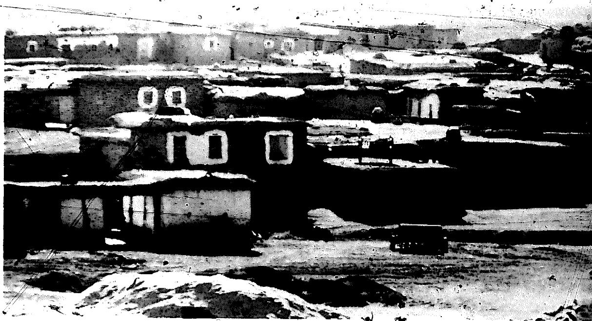
44 Rural housing in eastern Turkey. These homes are built of dried mud (adobe) with very heavy roofs, and the gap between houses is very small – a highly vulnerable set of conditions
