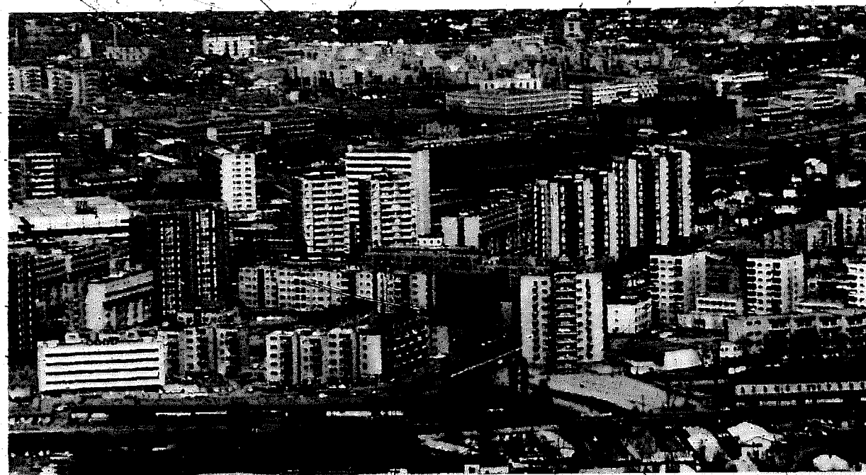
29 The central areas of Skopje, Yugoslavia, in 1975 - thirteen years after the earthquake
