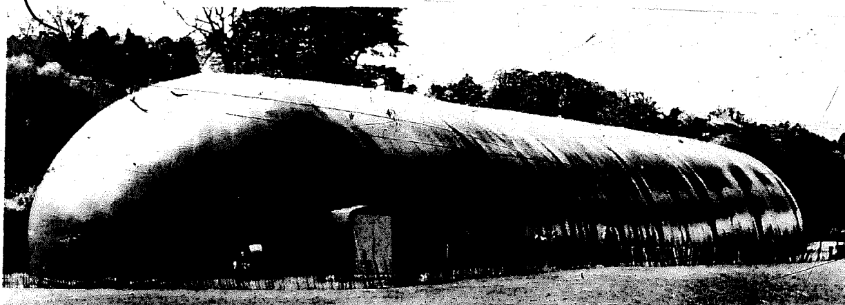
38 Inflatable grain warehouse. Proposals have been made for using such structures as emergency shelter
