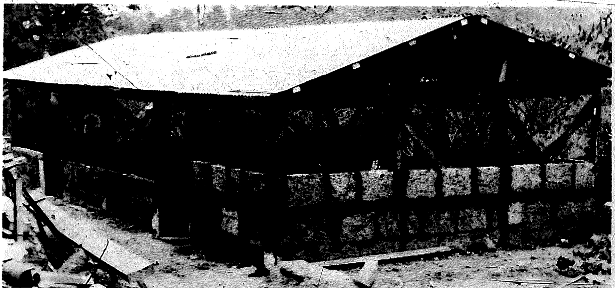
42 Model house built by Oxfam and World Neighbours, using safe construction techniques
