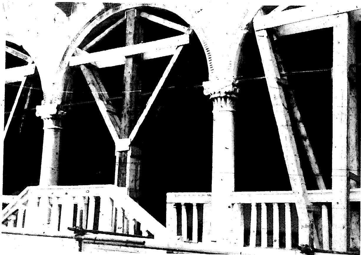
75 A shored-up arch in Gemona, Italy
