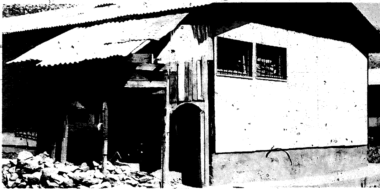
25 Prefabricated housing in Lice, Turkey, as modified by the occupants to give a protected front door and covering for animals
