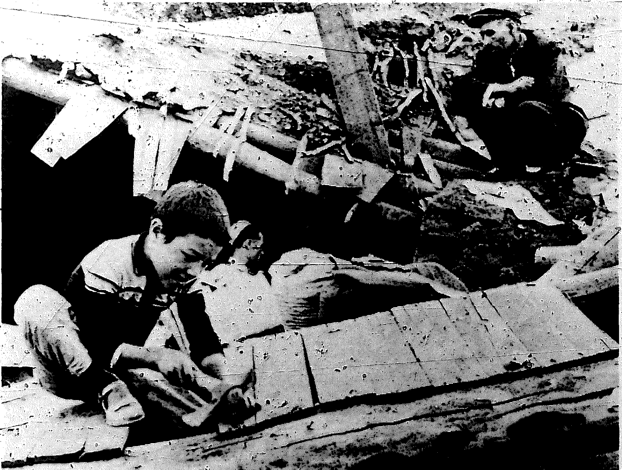
45 A family survey their wrecked home following the Turkish earthquake
