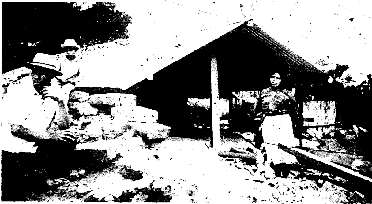
43 A new lightweight roof to replace the heavy tile roof which collapsed during the earthquake in Guatemala
