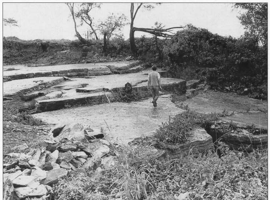
Figure 2: "Near horizontal layers of Rodeador marble, Minas Gerais, Brazil, showing Karstic rills on well developed joints"
