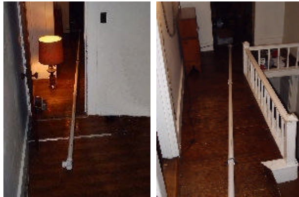
Bottom showing "T" fitting Mid- section showing guy bracket
