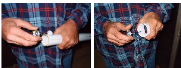
Apply glue to pipe Apply glue to coupling
