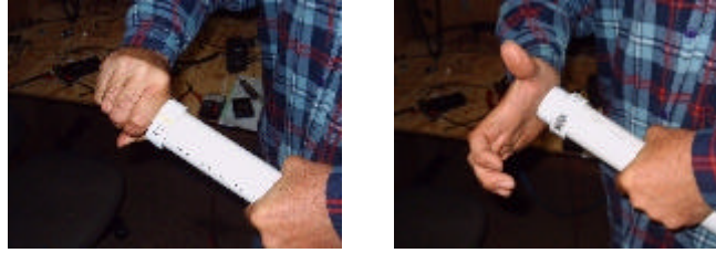
Twist coupling onto pipe Hit it with your hand to seat coupling
