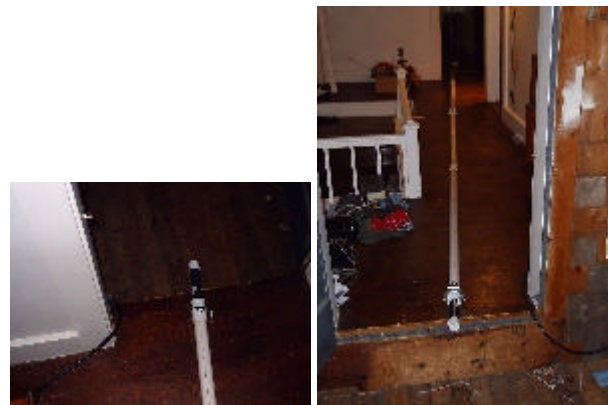
Bottom showing "T" fitting Mid- section showing guy bracket
