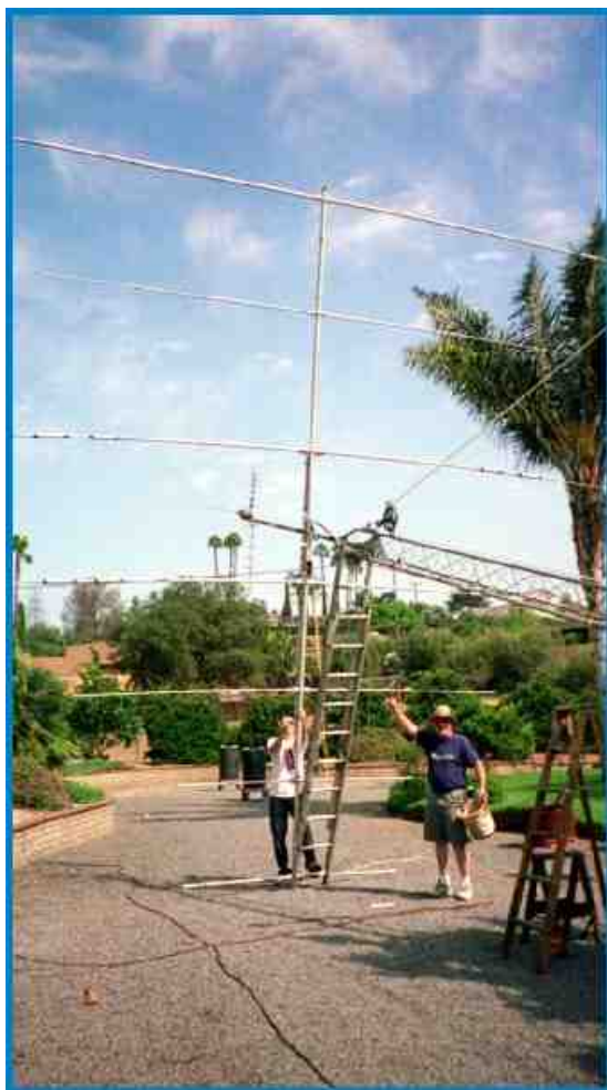
We used an extension ladder at the right height to support the tower and keep the antenna off the ground. The ladder is lashed to the tower and follows the tower as it is raised to this point.
