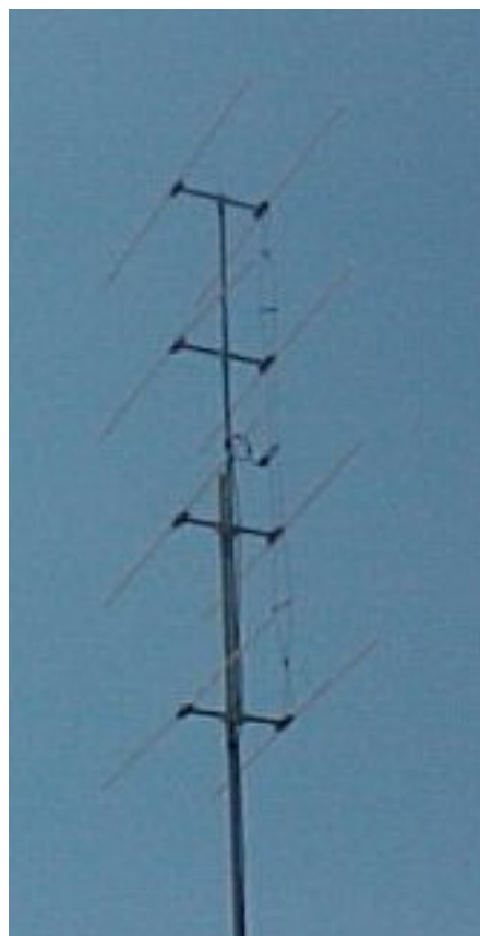
Figure 8. - four stacked half wave dipoles collinear antenna
