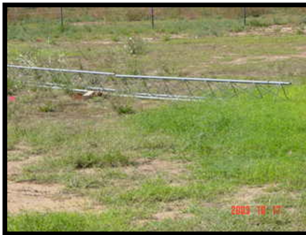
just south of the Crank up tower (see tower #1 page) Tower sections moved to location.
