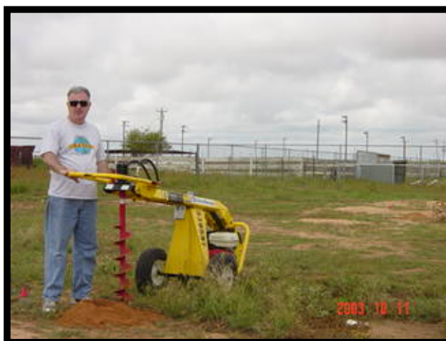
This is shot of project start.
