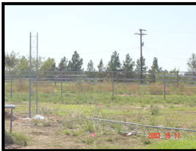
Hinged base. 1 st ten feet in place
