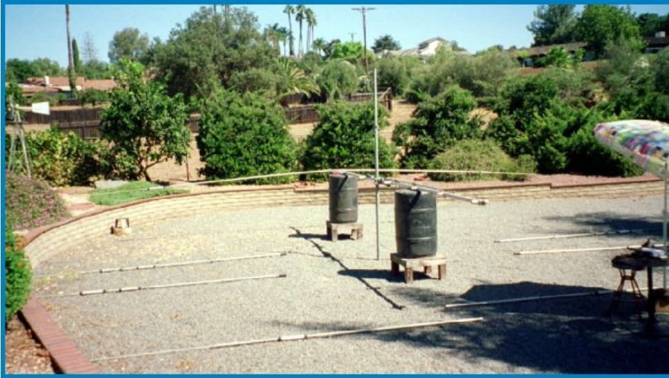
You need a level, elevated, surface to assemble this antenna. This is how I did mine.
