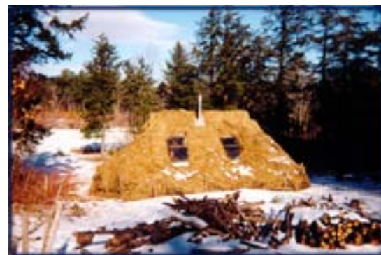
Student Housing. Students in the ESSP program stay in this shelter at the center of the Beartraks property.
