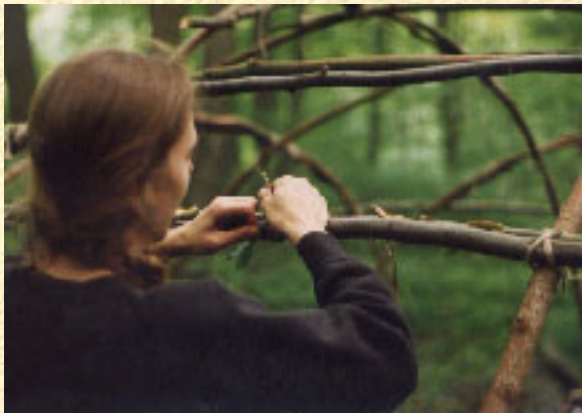
Me, lashing the hoops onto the wigwam poles, which gives the structure added support.
