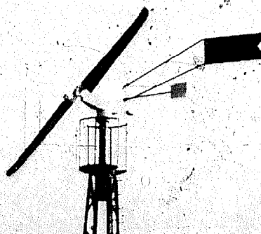
"Ideolec" Wind Generator
