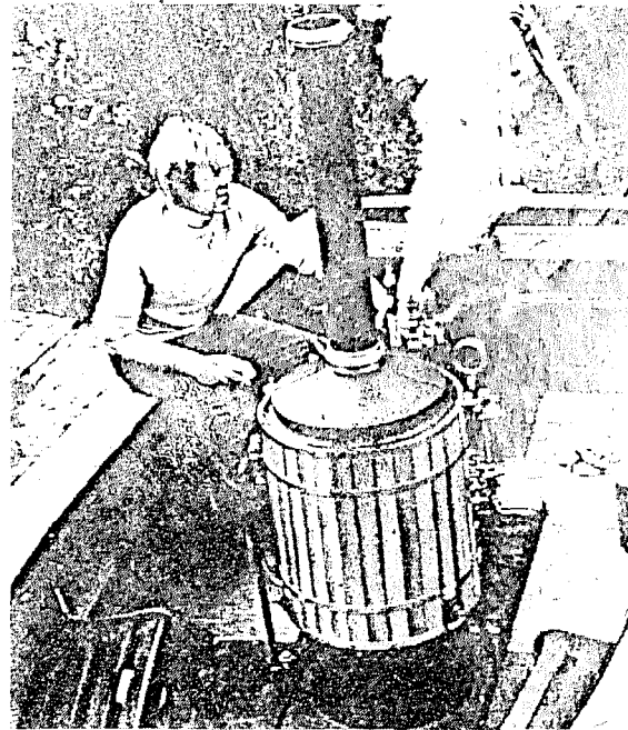
Vertical Coal Fired Boiler
