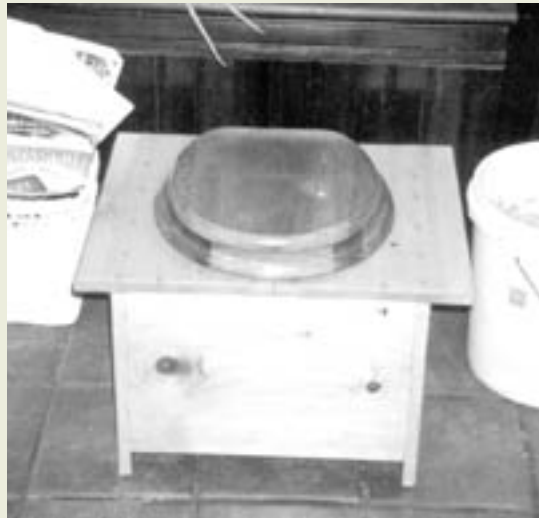
LIFT-OFF SAWDUST TOILET IN RURAL HOME
