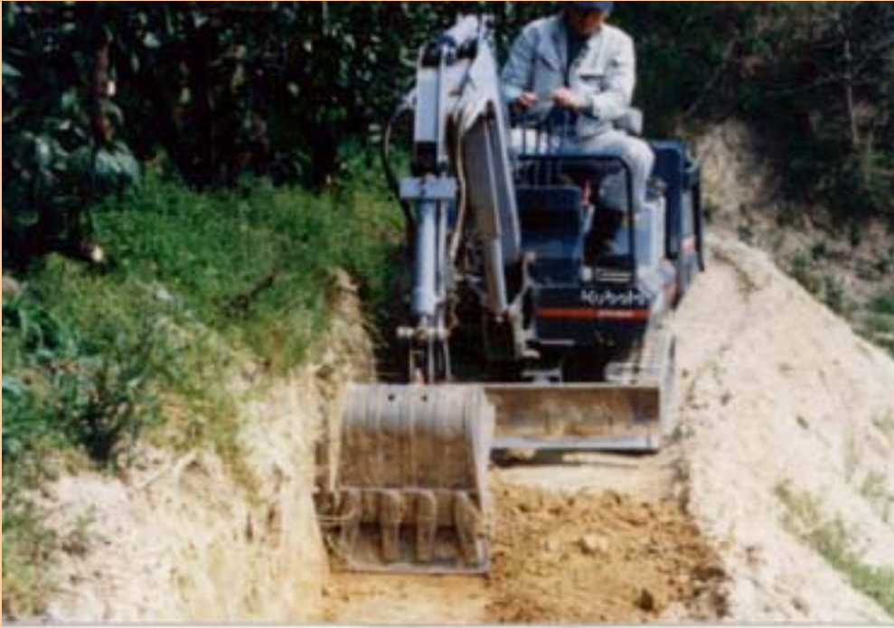
(1) Digging out using a small back hoe
