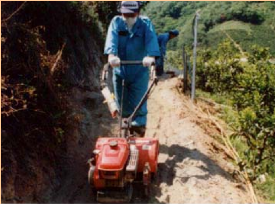
Fig.2. Construction process of farm path
