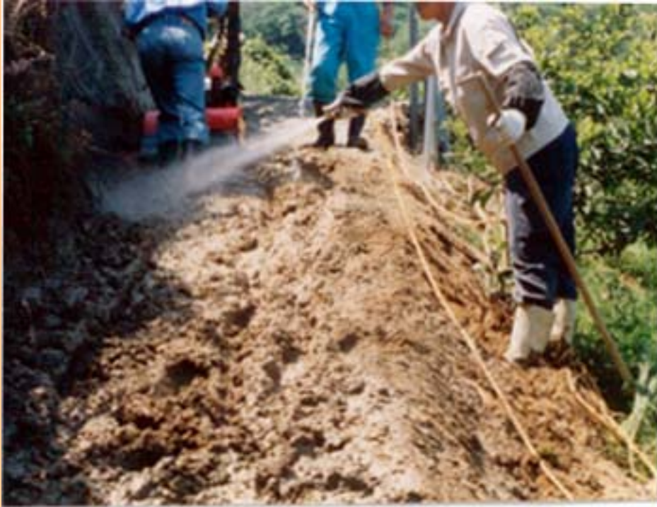
Fig.2. Construction process of farm path
