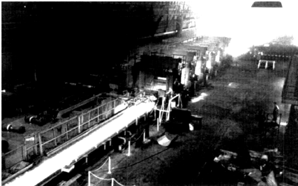
Figure 5.14 Hot strip finishing mill composed of 6 stands, each driven by a 2500 kW dc motor. The wide steel strip is delivered to the runout table (left foreground) driven by 161 dc motors, each rated 3 kW. (Courtesy of General Electric)
