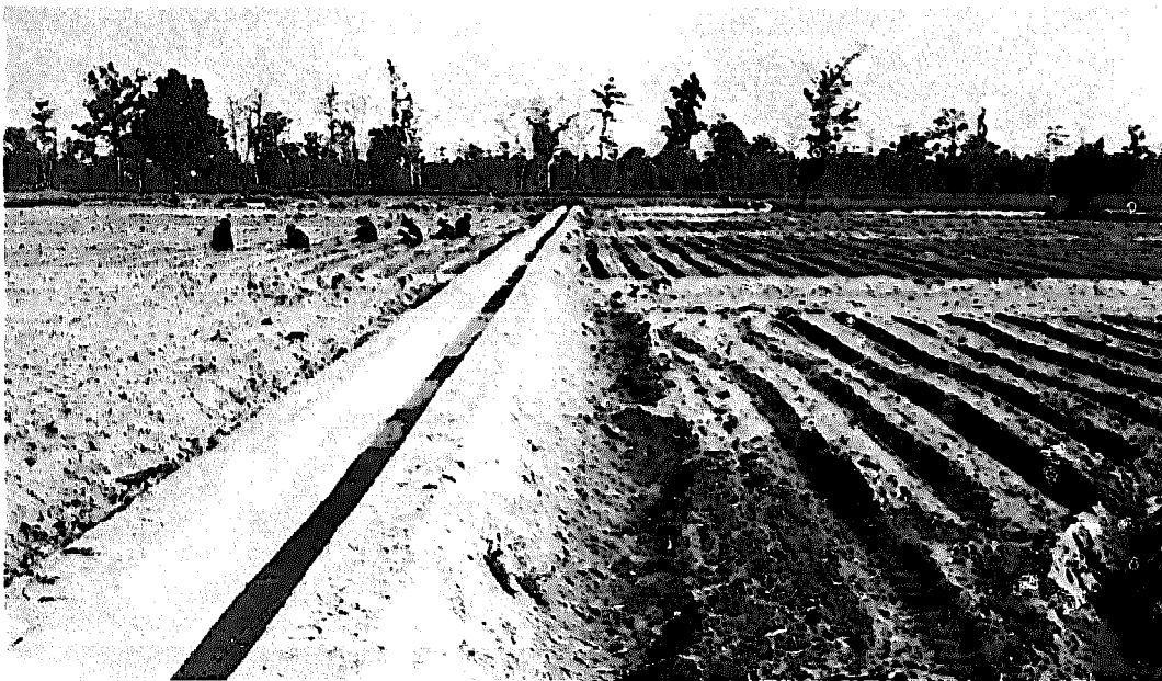
FIGURE 21. Concrete lining in elevated ditch supplying irrigation water to basin furrows.
