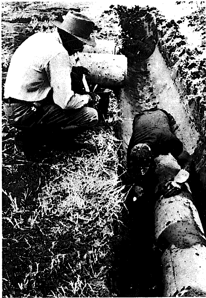
FIGURE 34. Workman installing precast concrete pipe in trench.
