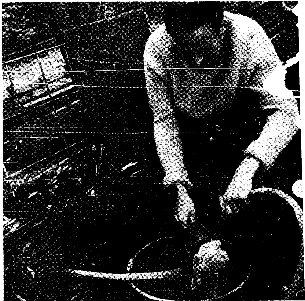
47. Small submersible electric pump for layflats
