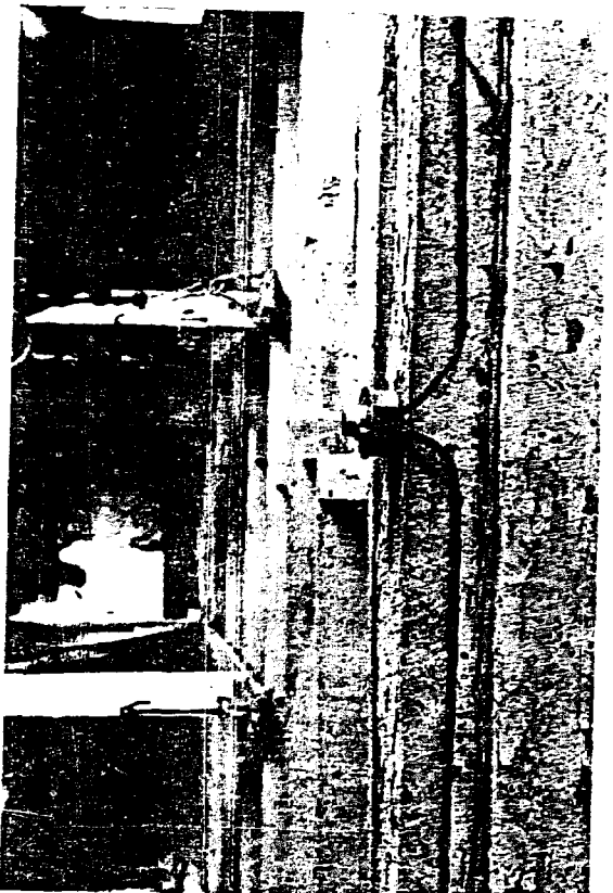
Figure 17. NON-METALLIC SHEATHED CABLE IN A DAIRY BARN.
