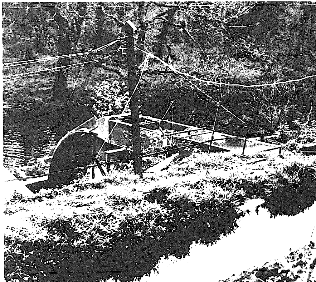
Photo 2 — The open channel takes water to the sluice gate where it enters the flume before filling the buckets on the wheel
