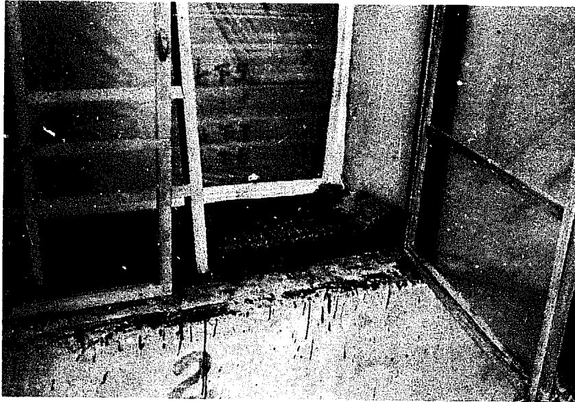
Photo 10 - Fibre mats dusted with chemical to prevent insects from entering when doors are open for ventilation (First Depot, Wuxi)
