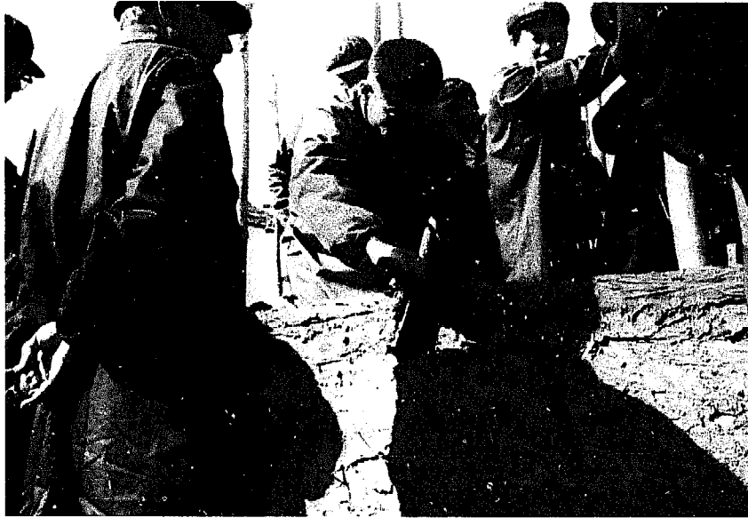
Photo 28 - Compaction and levelling of the wall are absolutely essential to arrive at high-quality wall. (Niou Pao Tin Depot)
