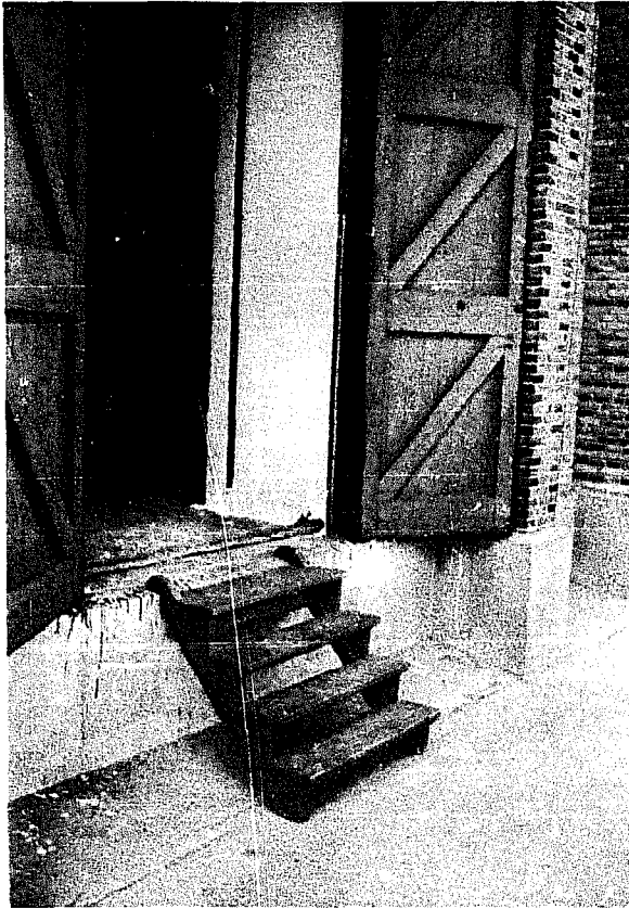
Photo 43 - Type "51" bulk grain warehouse. Floor level 0.60 m. Slot in pillar to fix plank wall to support grain pile. Fibre mat across the opening dusted with insecticide. (First Depot, Wuxi)
