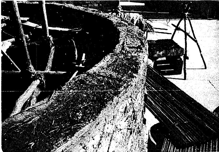
Photo 29 - 20 cm thick silo wall. Density of the clay/straw wall must be 966 \text{ g/cm}^3 or more.
