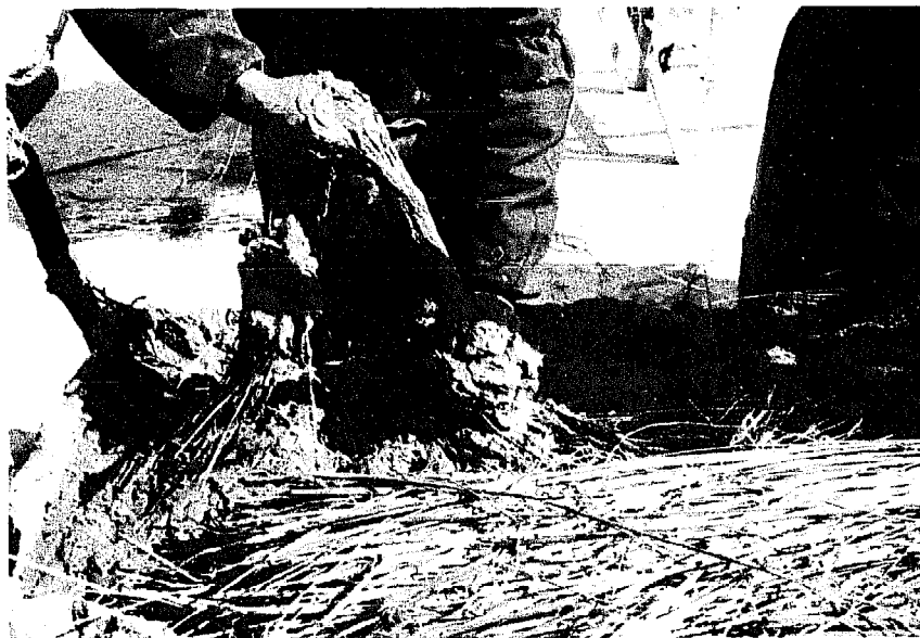
Photo 25 - When straw bundles are thoroughly covered with clay mud, excess mud is removed. (Niou Pao Tun Depot)
