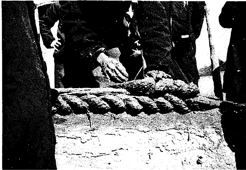
Photo 32 - Construction of eaves. The first layer has been placed and second layer is being started, with the clay/straw bundles turning in the opposite direction. (Niou Pao Tun Depot)
