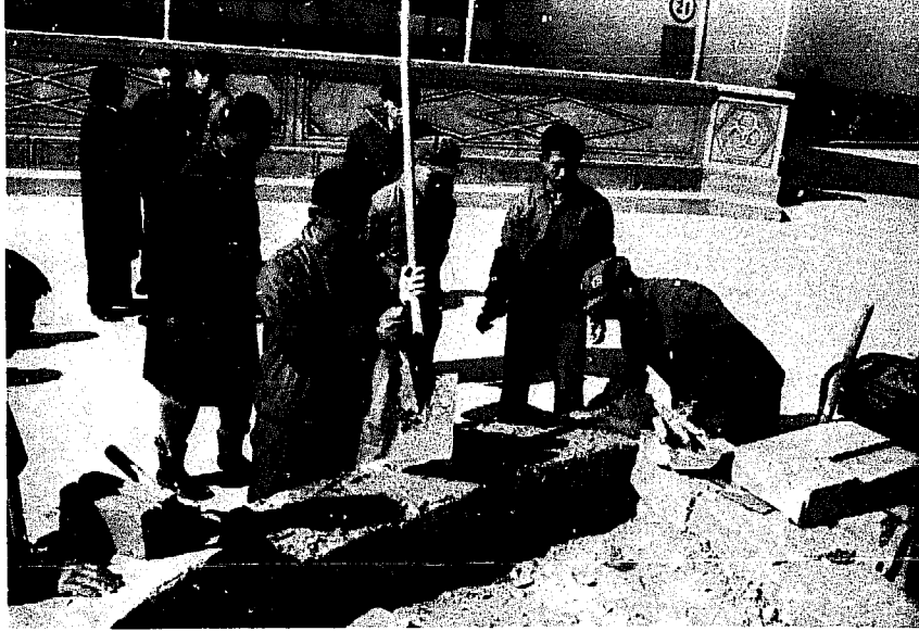
Photo 22 - Placing a brick layer on top of stone foundation wall (Niou Pao Tun Depot)
