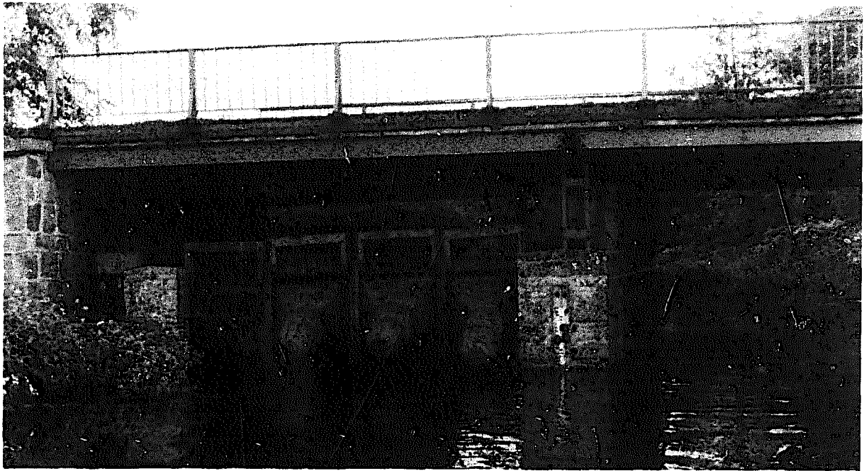
Fig 254 Permanent barrier in the river Eider in northern Germany at the outlet of a lake (Westensee), with baskets made of iron.
