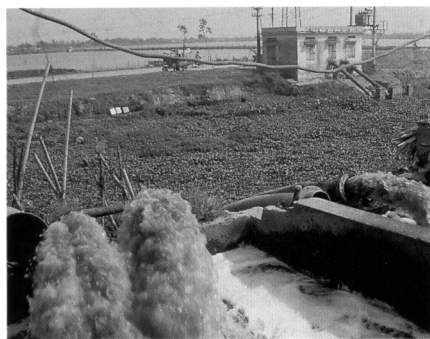
Pumping wastewater from Kim Nguu river
