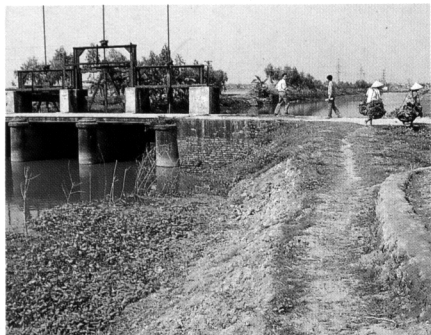
Water gate on Kim Nguu river
