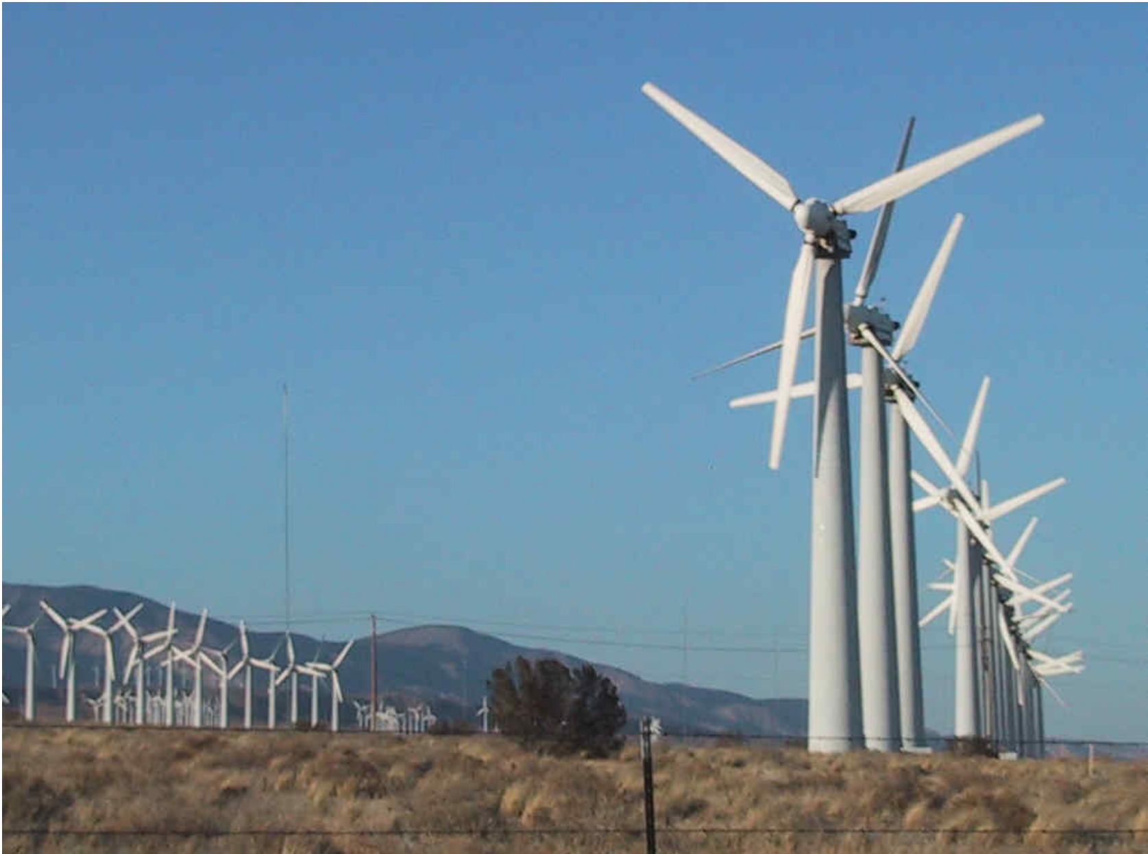
The Mitsubishi Heavy Industries Wind Farm, down the road. Row upon row of rotors, each with its own separate tower and generator.
