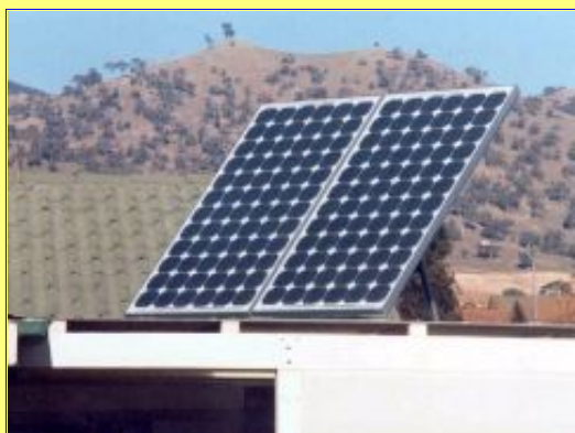
The solar panels on my roof. There are 2 more to come, for a total of 560 Watts.
