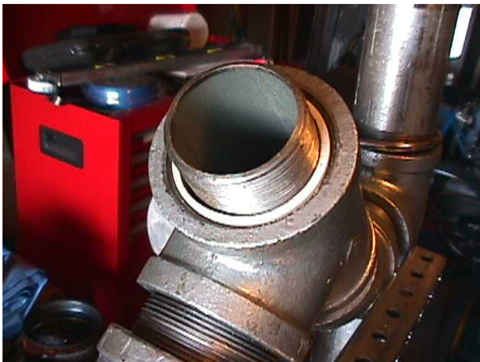
Note the PVC bushing on the inside of the furling pipe.
