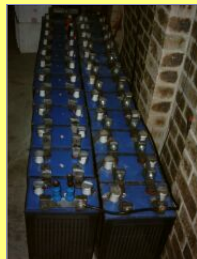
The whole battery bank - 1100Ah at 24V. Total weight ~ 1500kg.
