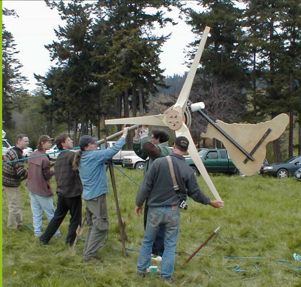
Putting the larger machine onto the tower for erection. The tail is a map of the island.
