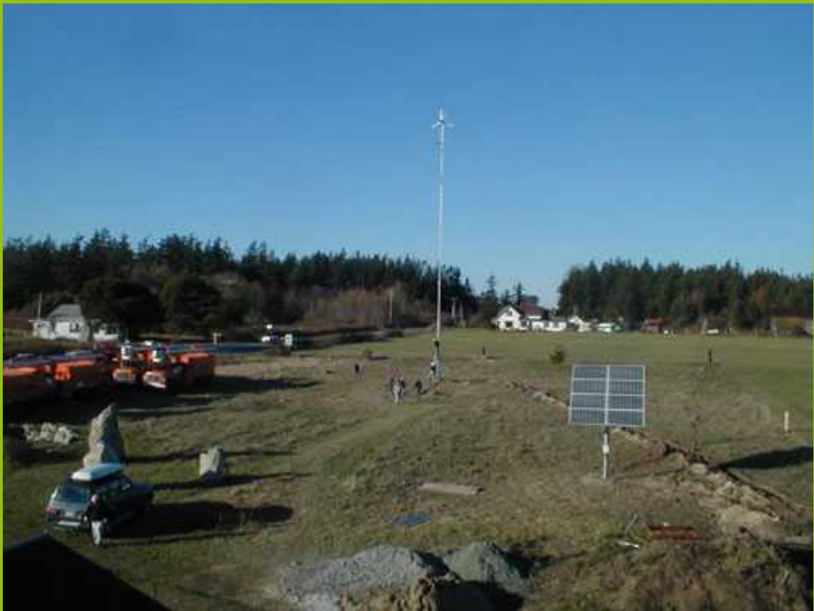
Here is the power room with the SW inverter that manages the inertia.
