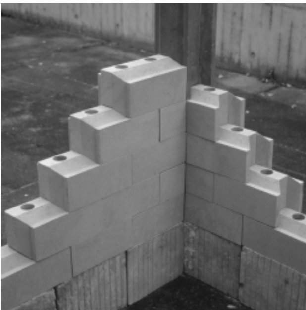
7-15 Improved interlocking system of FEB, Kassel, 2001
