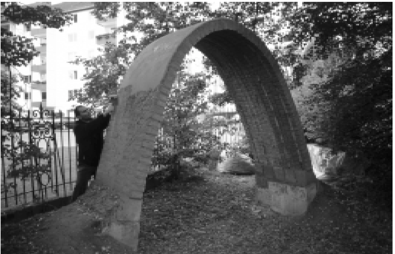
15-7 Construction of the arc with split bamboo
