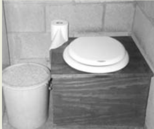
EMERGENCY SAWDUST TOILET IN BASEMENT OF NEW HOME WITH SEPTIC SYSTEM
