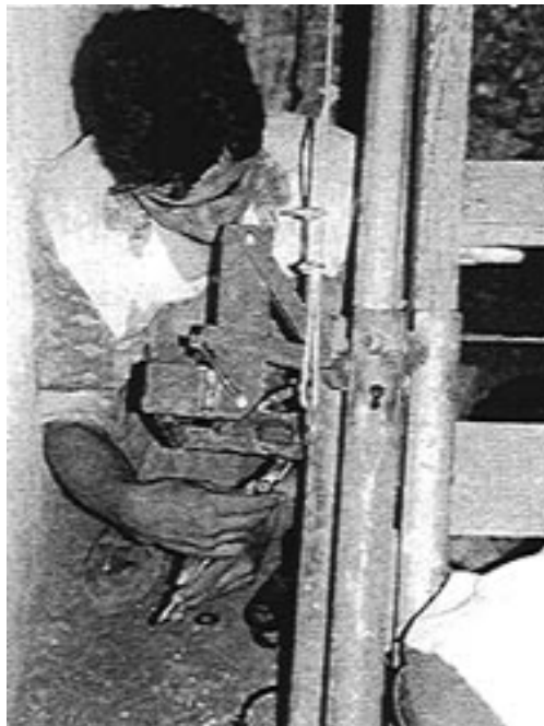
Marcelo installs the safety latch.
