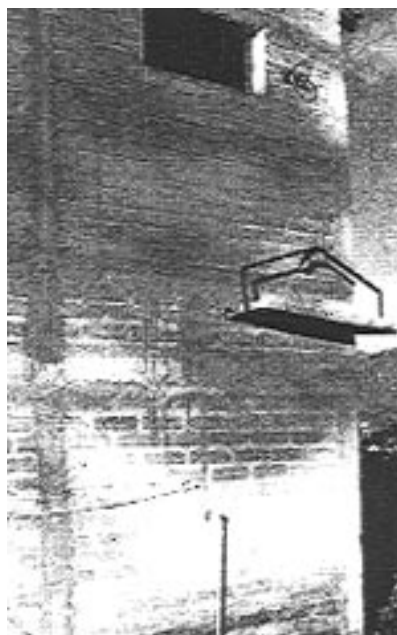
The counter-balance on the outside wall is weighted with cement blocks.
