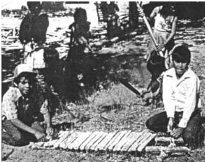
Out of poles they collected from the local forest, school children make a ramp as part of the equipment for the playground.
