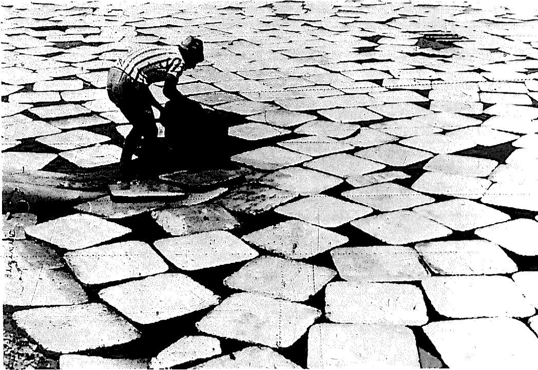
FIGURE 42 Protective covering of molded, lightweight, concrete slabs cut evaporation by an estimated 80 percent recently in full-scale tests on two reservoirs in Ovamboland, South-West Africa. Engineers cover reservoirs with 24-in 2 , 2-in thick floating slabs of polystyrene, sand, and concrete. Exposed surface of each slab is painted white to reflect the intense sun rays, which hasten evaporation.
