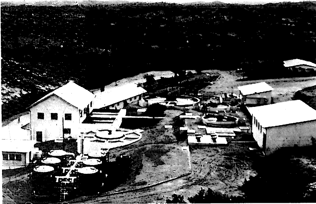
FIGURE 32 City of Windhoek, South-West Africa, (population 84,000) on the edge of the Namib Desert cycles its municipal wastewater through this treatment plant and back into the potable supply. (National Institute for Water Research, Pretoria, South Africa)
