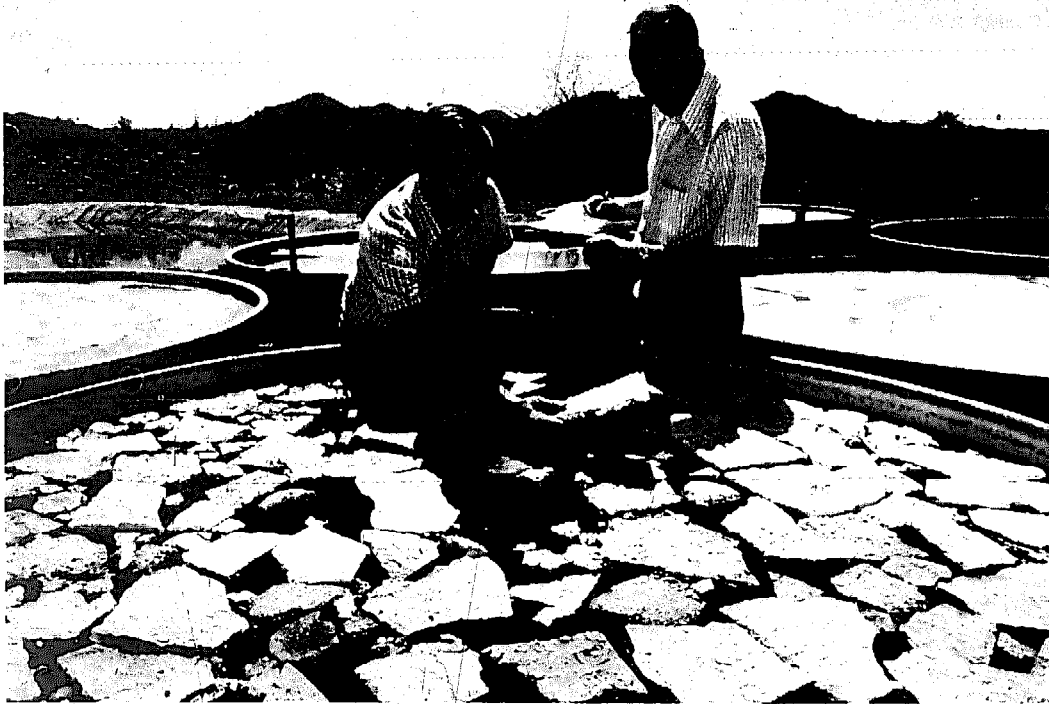
FIGURE 41 An experiment in Arizona, USA, using wax to suppress evaporation. Blocks of wax have been added to the tank (foreground). Sun's heat melts the wax to form the continuous film visible on the tanks in the background. During 4 years this film has suppressed over 85 percent of the normal evaporation. (K.C. Cooley)
