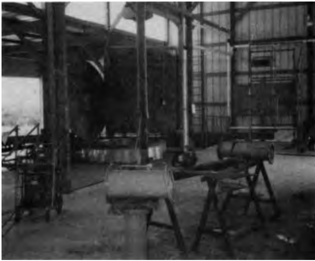
Texarome distillation plant for extracting natural oils. Courtesy of Texarome, Leakey, Texas. (SFP-13)
