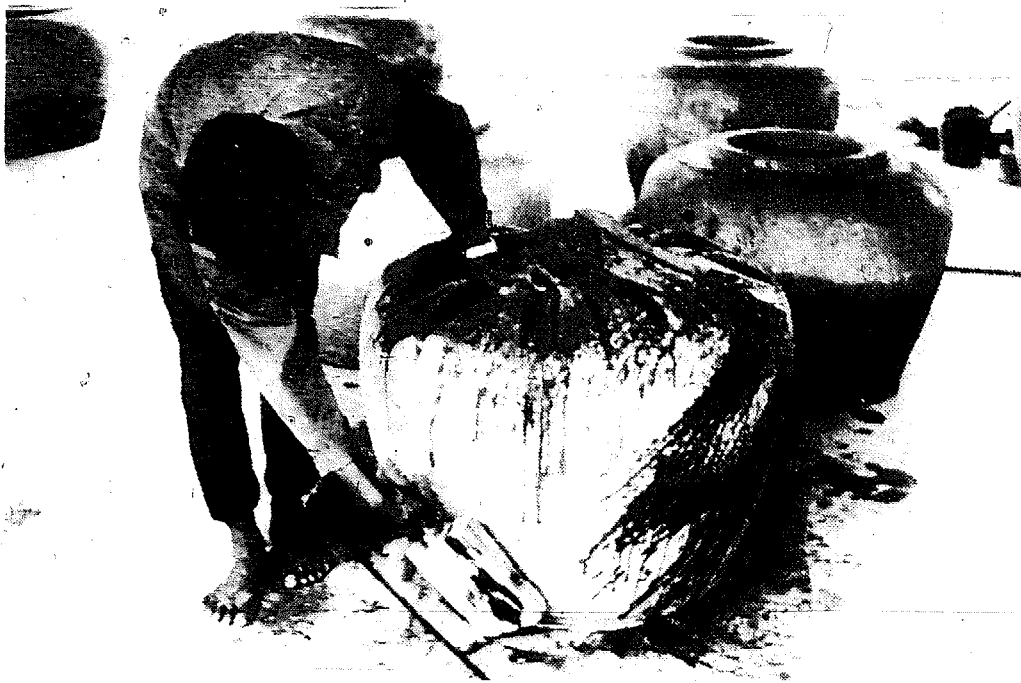
2.5 When the sack is filled up, fold the top and tie it into the shape of a traditional water jar. Use a piece of wood to tap on the mould to make it round and fair.
