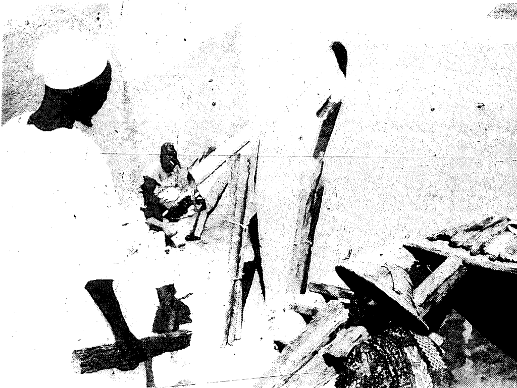
7.6 Building the roof; bottom right
