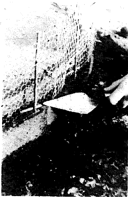
5.4 Bend up reinforcement
