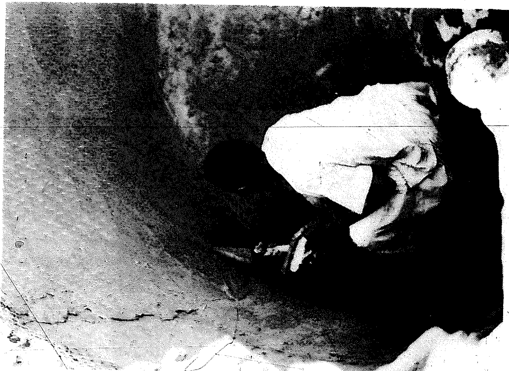
7.3 Lining tank with chicken mesh and mortar
