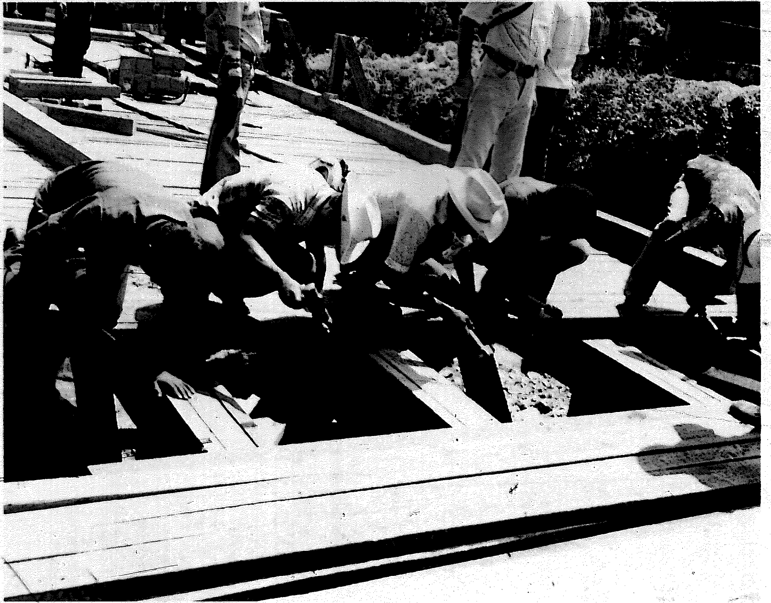
Completing the nail-laminated deck, Honduras
