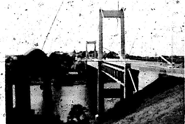
Fig 1.22 Brunei's bowstring girder bridge of 1839 and the Saltash suspension bridge at Budeaux, Plymouth
