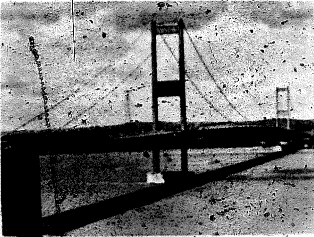
Fig 1.24 The Severn bridge. This has a main span of just under 1000ft. Together with the bridge over the River Wye, this 18 000 000 bridge forms part of the M4 motorway from London to South Wales.
