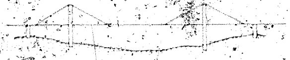
Fig 1.26 The Wye bridge is of the stayed girder type, a design new to this country, applying what is, in effect, the cantilever principle in cable form.
