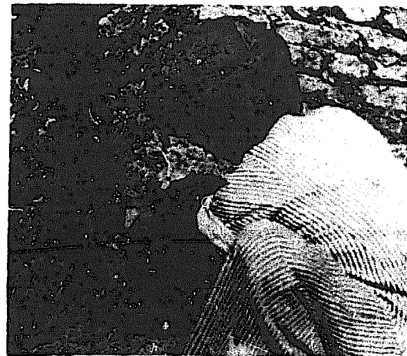
FIGURE 6. A mason is placing the first brick. This first brick is very important, as it sets the cant of the remaining brick courses in the vault. The mason has placed this brick almost flat against the end wall. The base which is resting on the side wall is about one inch from the end wall. The top of the brick rests against the end wall. This gives a slope to the brick courses of about 1 to 10. This brick is held in place by mud mortar and friction developed by small grooves on the back face of the brick. It has its main thrust downward which is carried by the side wall. The brick also has some horizontal thrust which is taken by the end wall.
