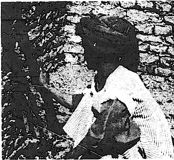
FIGURE 10. The mason is applying the mud mortar for the next course. Some masons have trowels, but most of the masons in upper Egypt use their hands as trowels.
