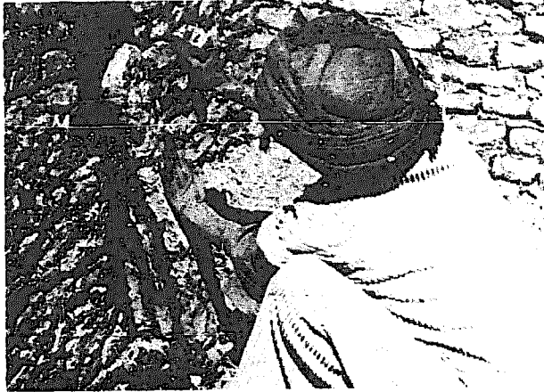
FIGURE 9. The mason is tapping the third and final brick in the third course. The cant of the vault is now beginning to be noticeable.
