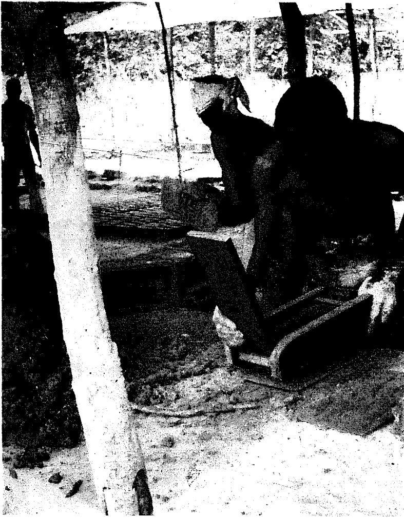
Alternative system using single self-releasing mould in conjunction with the sandmoulding method
