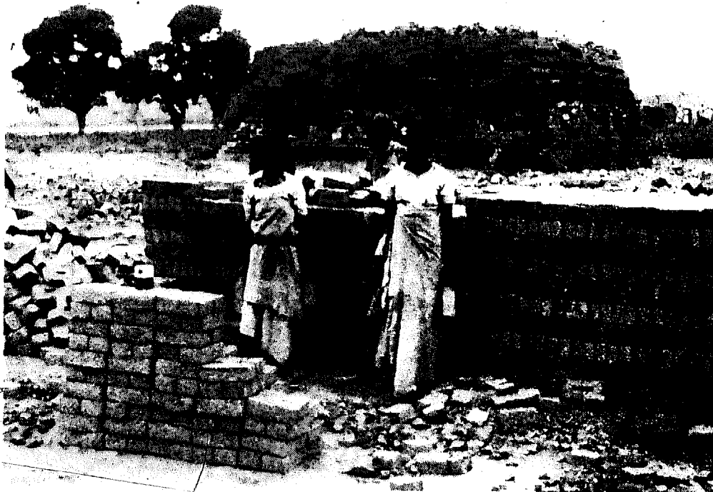
Wood-fired clamp under construction by lady brickmakers. Lack of suitable hand trucks leads to excessive carrying. Some shape defects can be seen in bricks in the foreground
