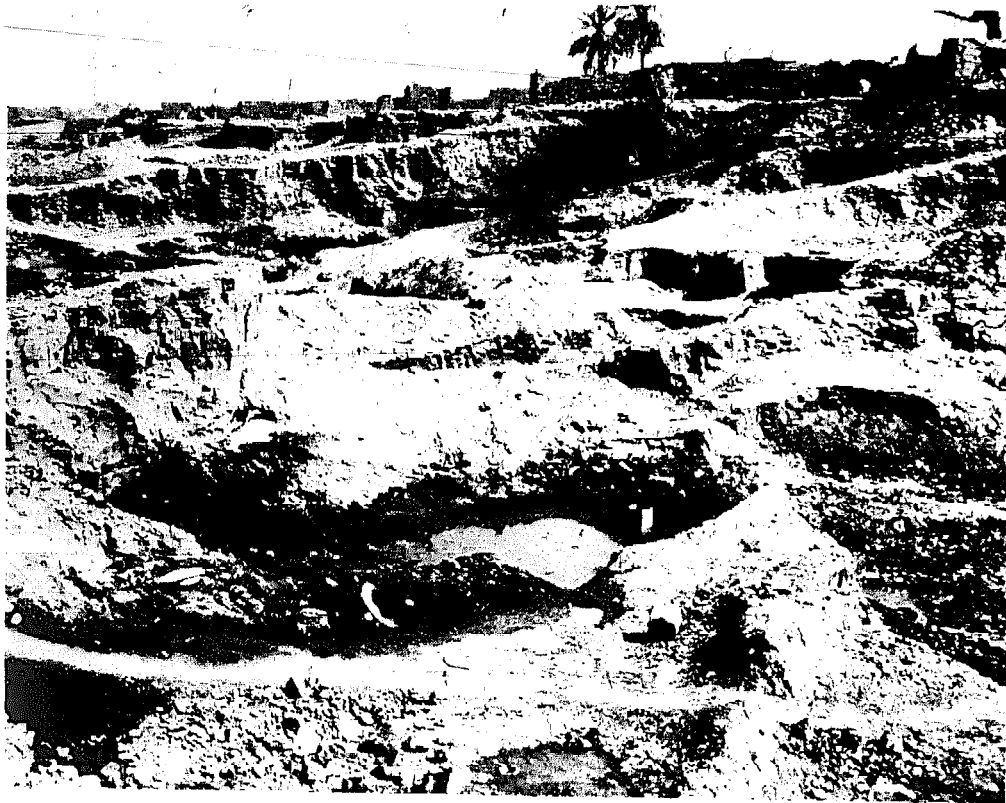
Clay dug and mixed with water, straw and camel dung at the river bank
