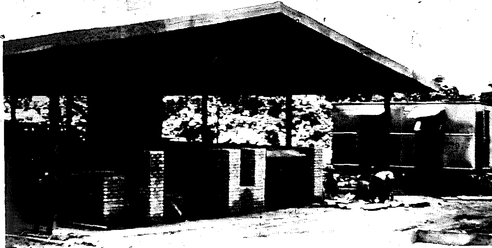
An originally constructed, side-fired double chamber kiln specially designed for wood firing, in use at Asokwa and Ankaful brickworks. Fuel consumption was high because the kiln is intermittent and no heat is re-used from the bricks cooling down from previous fire. Subsequent measures applied to increase the height of the side walls are understood to have improved efficiency
