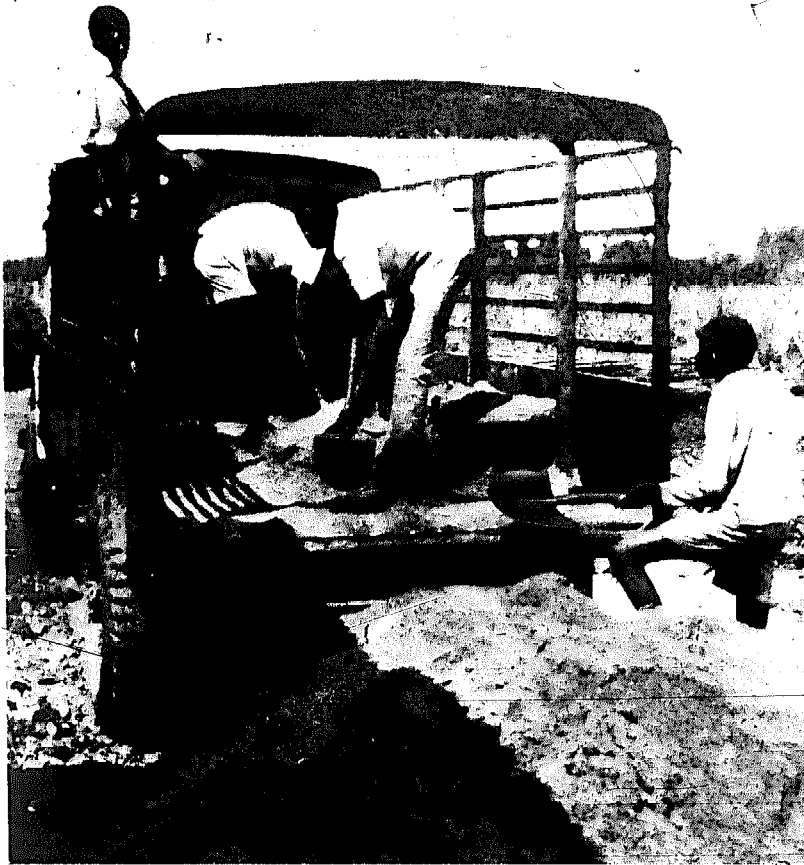
Additional cost incurred bringing sand to the brickmaking site if sand is not available in same location
