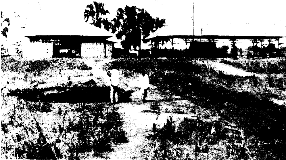
More expensively constructed brickworks with two production buildings
