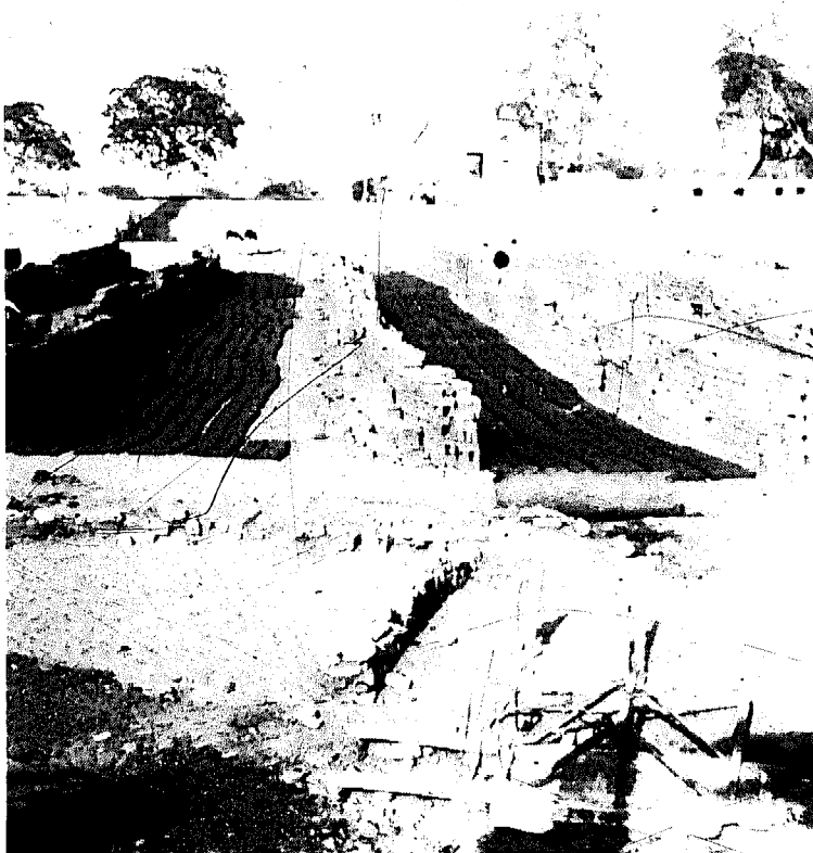
Bricks moulded onto the ground in extensive open working and drying area adjacent to kiln
