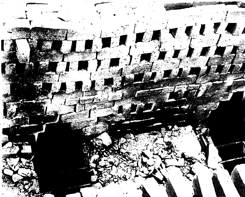
Firing channels act as hearth under setting, often producing more consistent results than large "tunnels" through the brick setting itself
