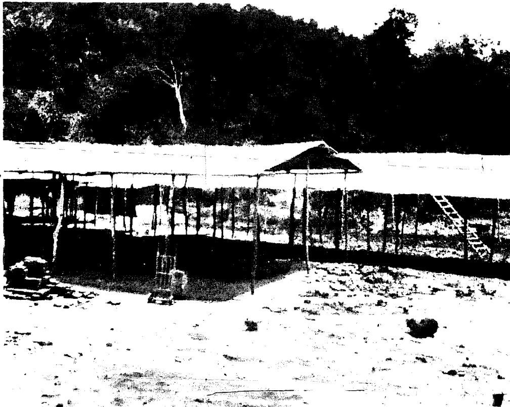
Corrugated-iron roofed working and drying sheds constructed out of rough timber cut from adjacent forest. Buildings need provision to adjust for different ambient drying conditions
