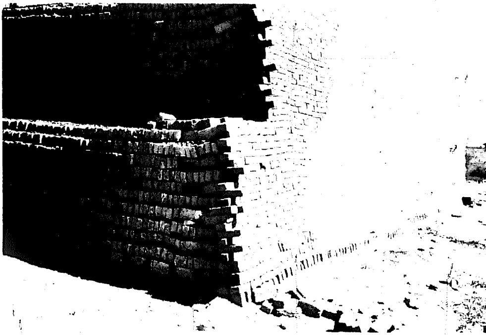
Extremely high standard of coal fired clamp construction likely to achieve a high efficiency of fuel consumption and consistent burning
