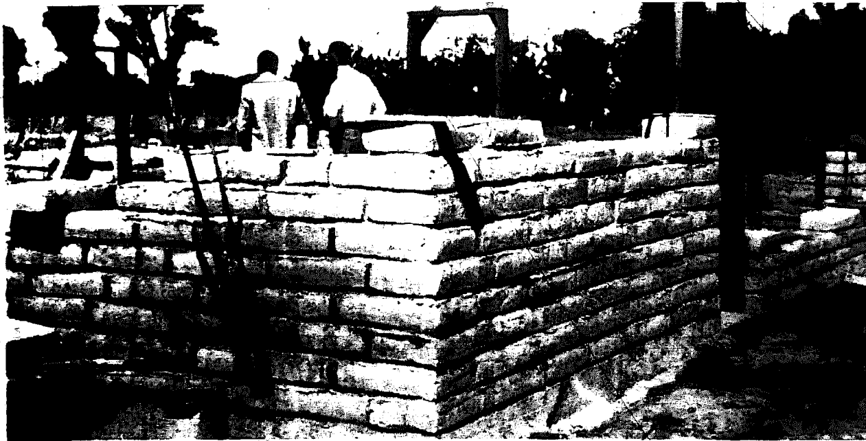
ADOBE-HOUSE CONSTRUCTION, showing brick arrangement, vertical reinforcing steel, and door frames in place.
