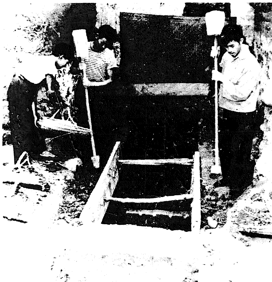
Plate 4-3. Pounding the walls firmly in making a rectangular pit of triple concrete.
