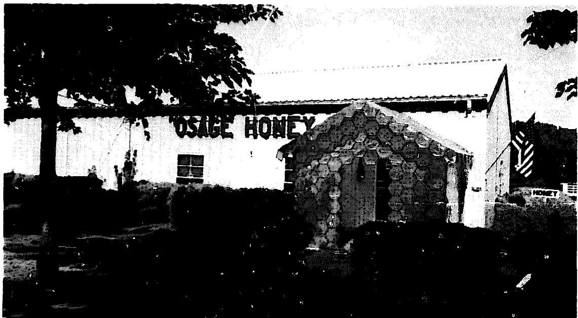
The all-metal honey house of Osage Honey Farms, Sibley Missouri. All steel buildings have the advantage of pre fabrication, can be assembled at the site. The entire building is insulated.
