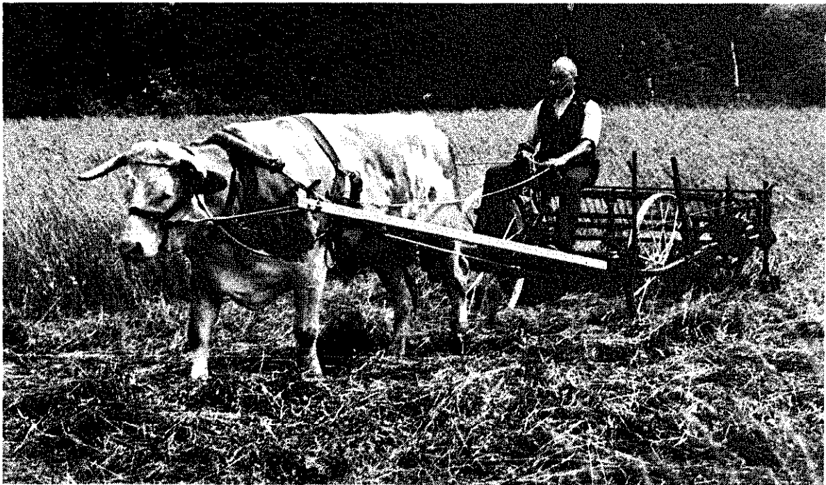
Fig. B/II/54 : Rake to be drawn by one or more animals: the direction of rotation of the swath cylinder can be reversed, making the implement suitable for turning and windrowing harvested crops. Note the precise harnessing using a halter and an individual withers harness. (Source: FAHR)
