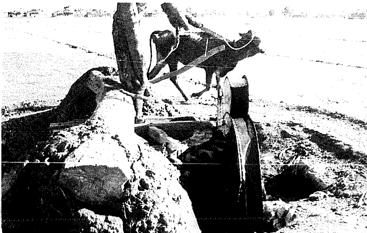
Fig. B/11/66: Continuous delivery of water using a bucket wheel. (Photo: GTZ Archives)
